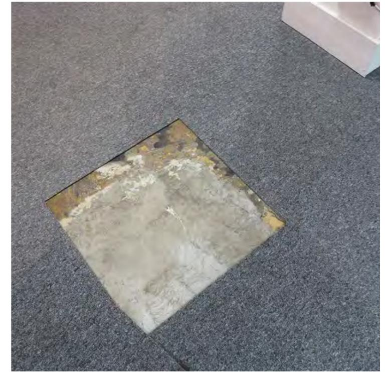
Existing modern carpet laid on screed which is in poor condition.
