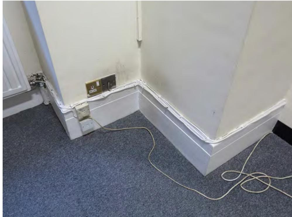
Existing wiring tied to walls. Some data and power chased into the walls.
