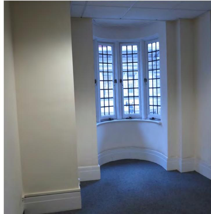
Historic windows and skirting. Large pilasters are new concrete blockwork additions, assumed for structural stability when the 5th floor was reconfigured.
