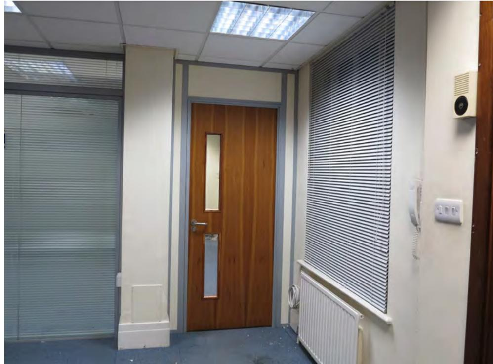
All doors are modern additions. Columns are steel I-columns clad in modern plasterboard.
