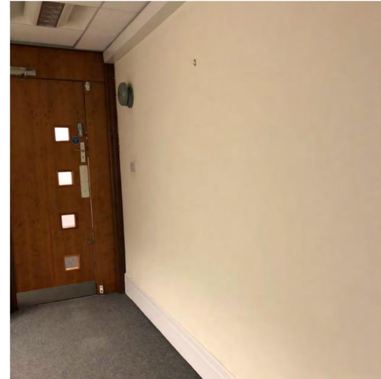
Historic structural wall along the centre of the floor plate. All doors, ceiling, floor finishes are modern additions
