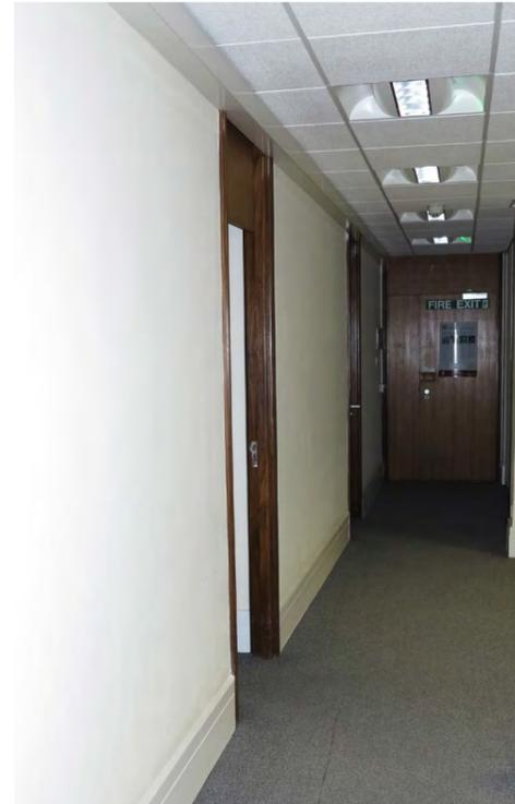
Historic structural wall along the centre of the floor plate. All doors, ceiling, floor finishes are modern additions
