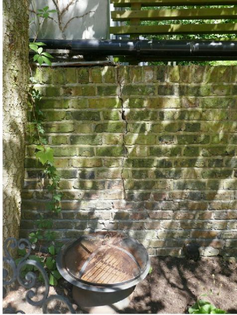
3) Crack in the wall near the outbuilding, trunk of the tree to the left.
