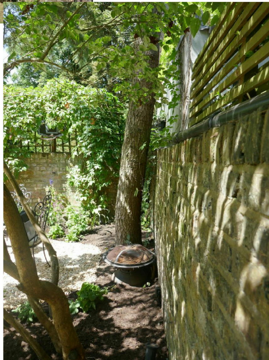
2) View along the wall towards the tree showing lean in the wall and trunk. White structure is the outbuilding at no.34.
