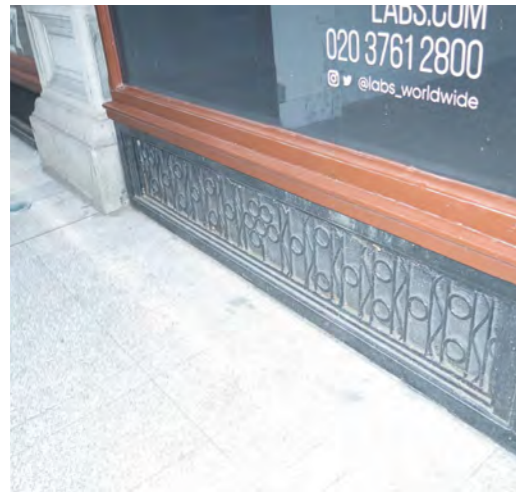
Unit 11 metal grille detail
