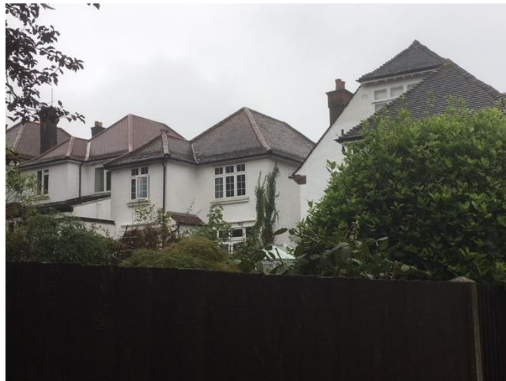
Rear of 35HW as seen from Langbourne Avenue
