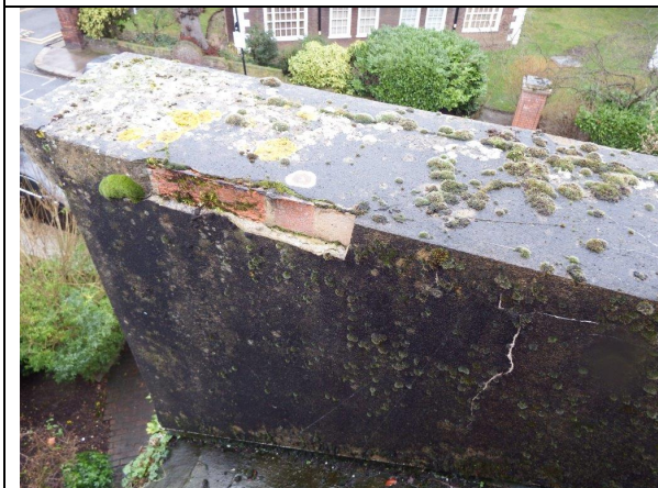
Parapet Walls Need Overhaul
