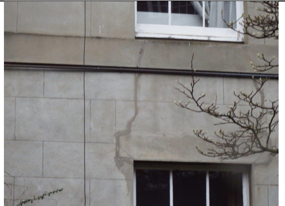
Cracks to Render
