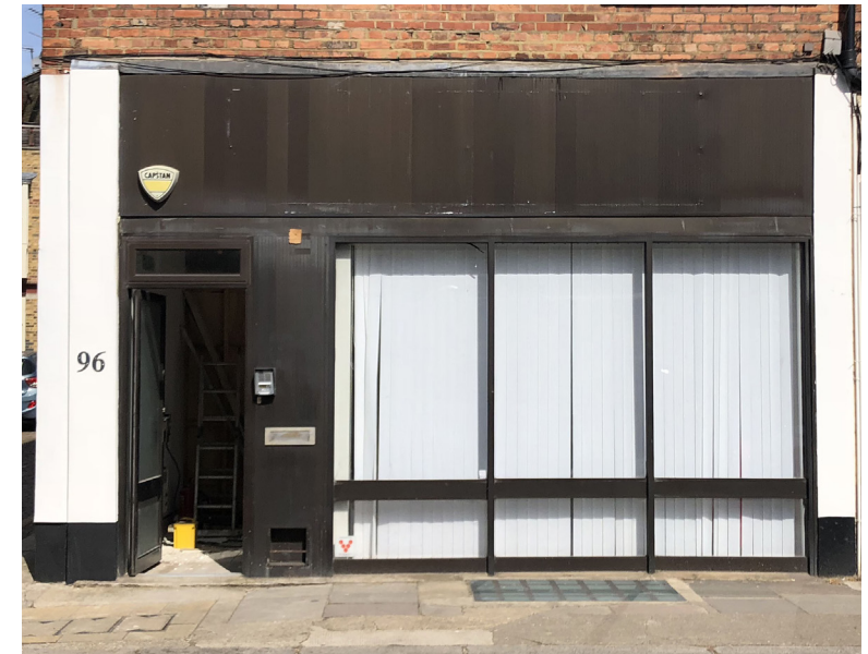
1) Existing shop front
