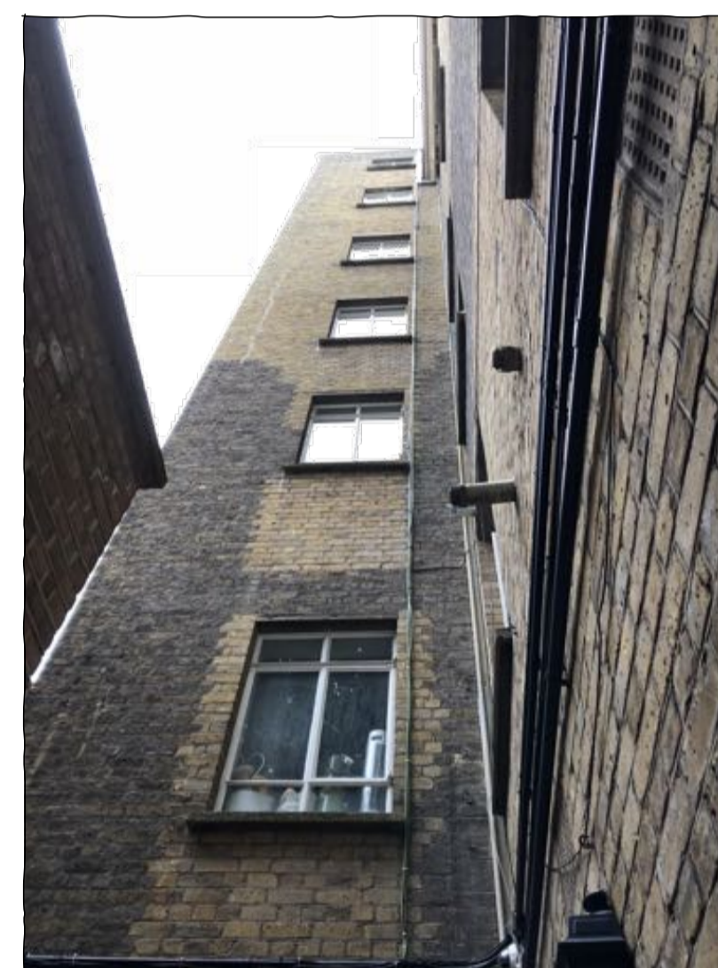
photograph A taken from basement ground level
