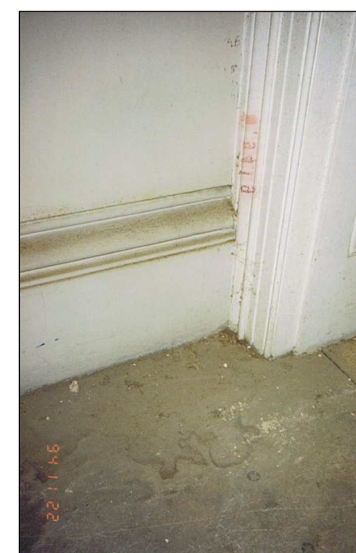
Reference photograph from 1994 - 9 Cambridge Gate reference skirting type 1
