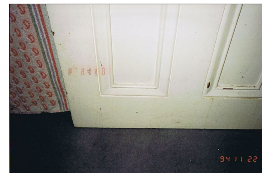
Reference photograph from 1994 - 9 Cambridge Gate reference door panels
