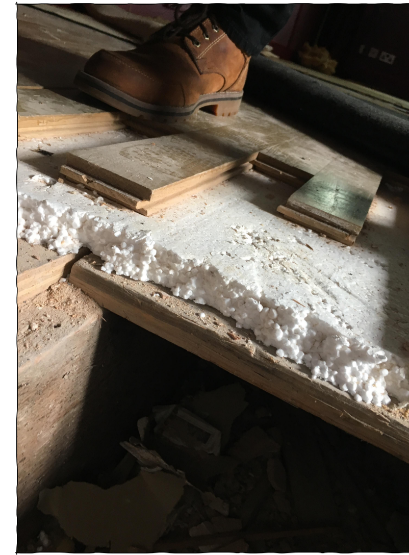
Typical existing floor makeup to be replaced
