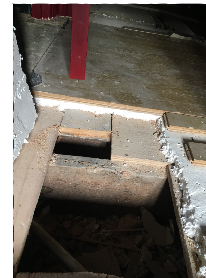
Typical existing floor makeup to be replaced
