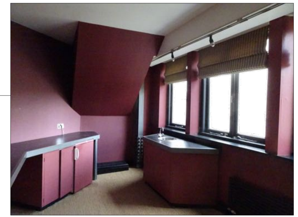
joinery, fixtures, fittings and enclosure stair partition and floor finishes removed
