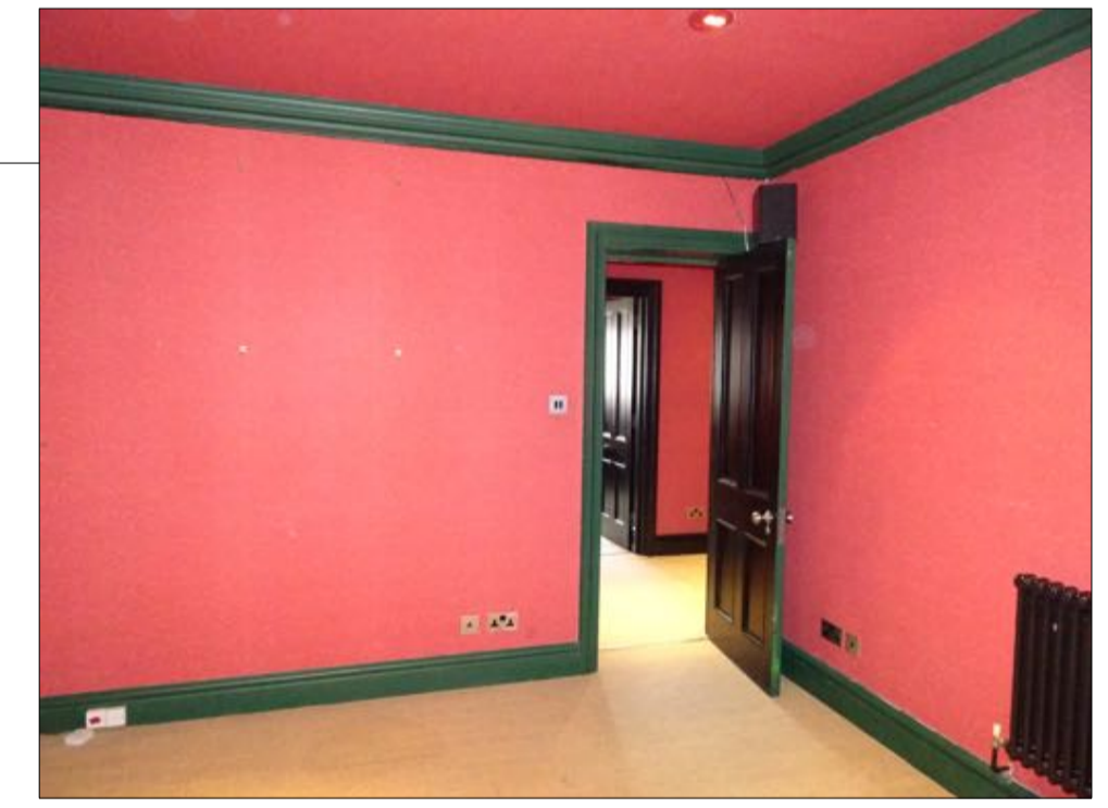
doors, skirtings, architrave, floor finishes and partitions removed
