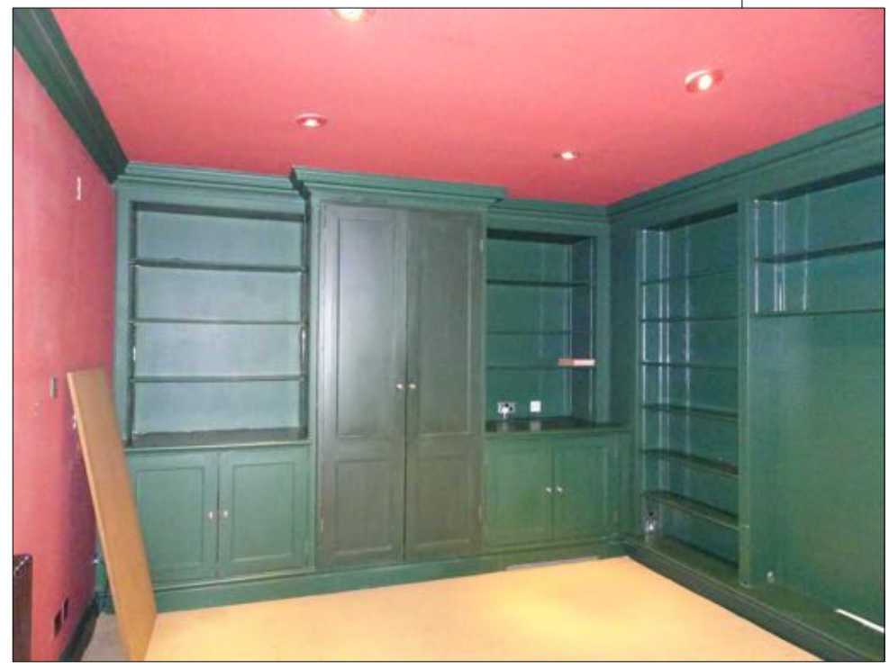
joinery, skirtings and corning removed
