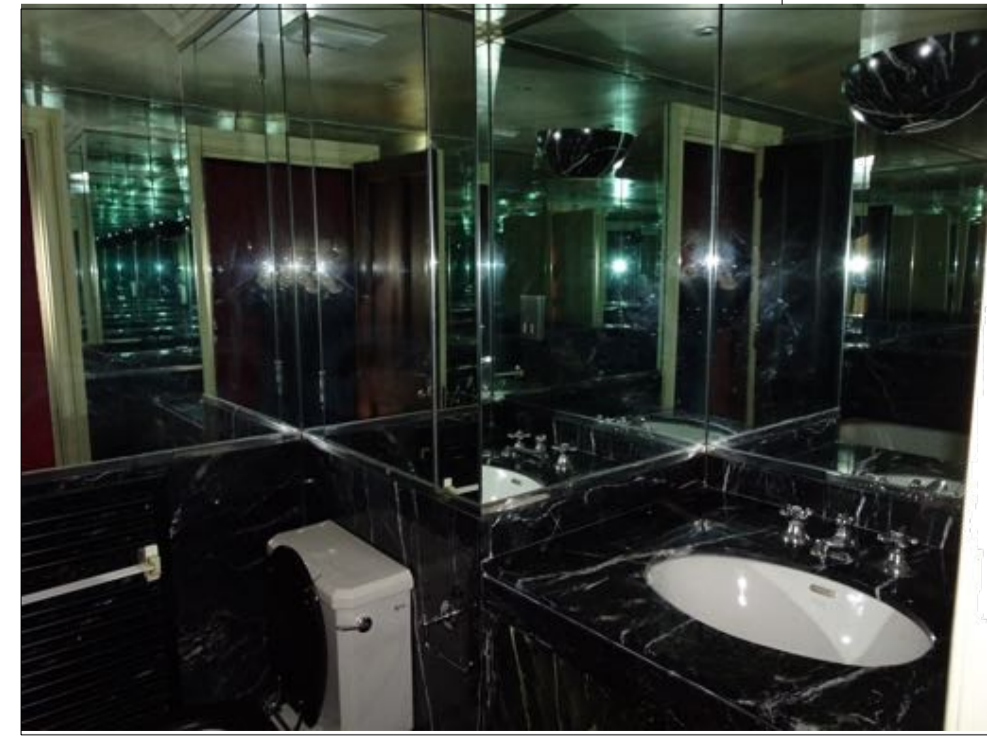
cloak room fixtures, fittings, services and joinery to be removed
