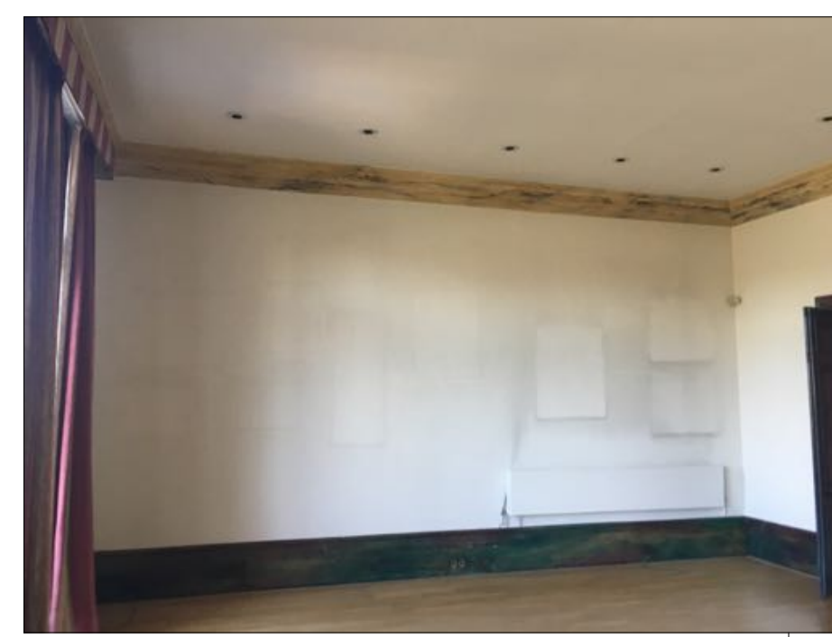
cornice skirtings and architrave removed
