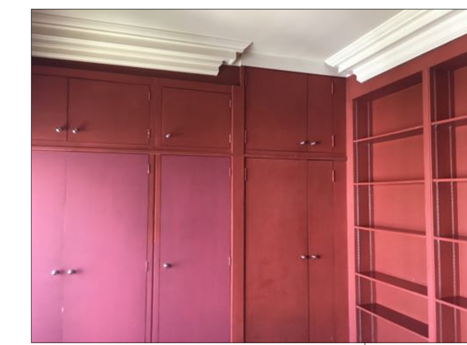
closets and cornice removed
