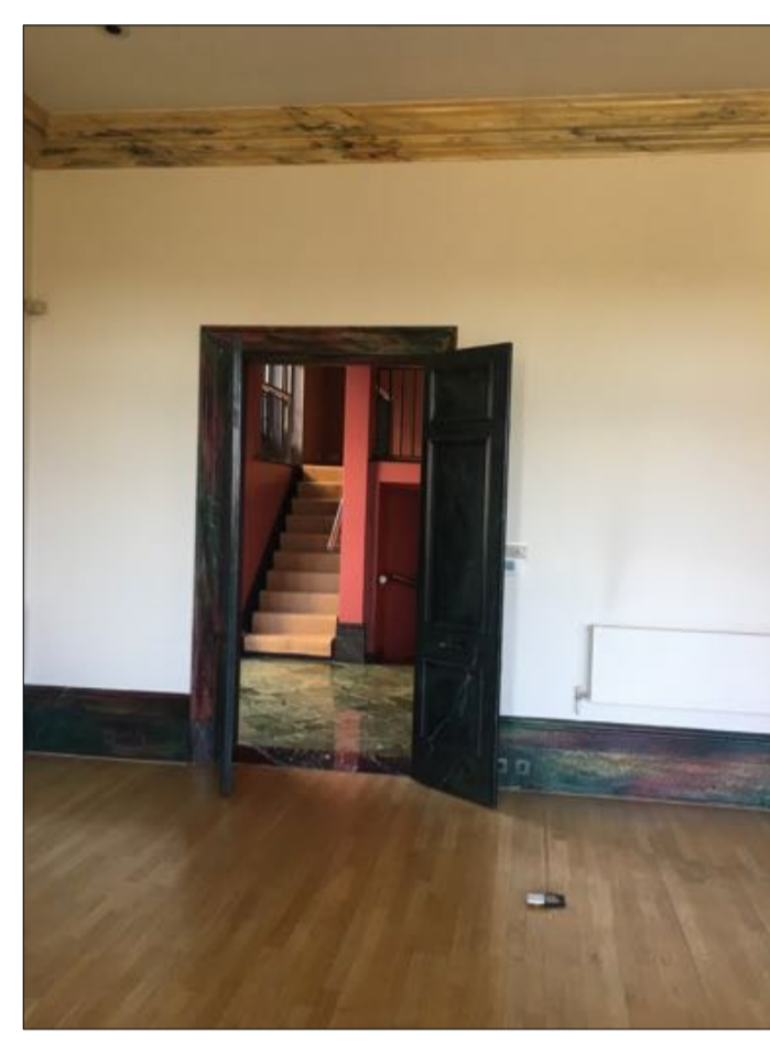
doors, skirtings, architrave and floor finishes removed.
