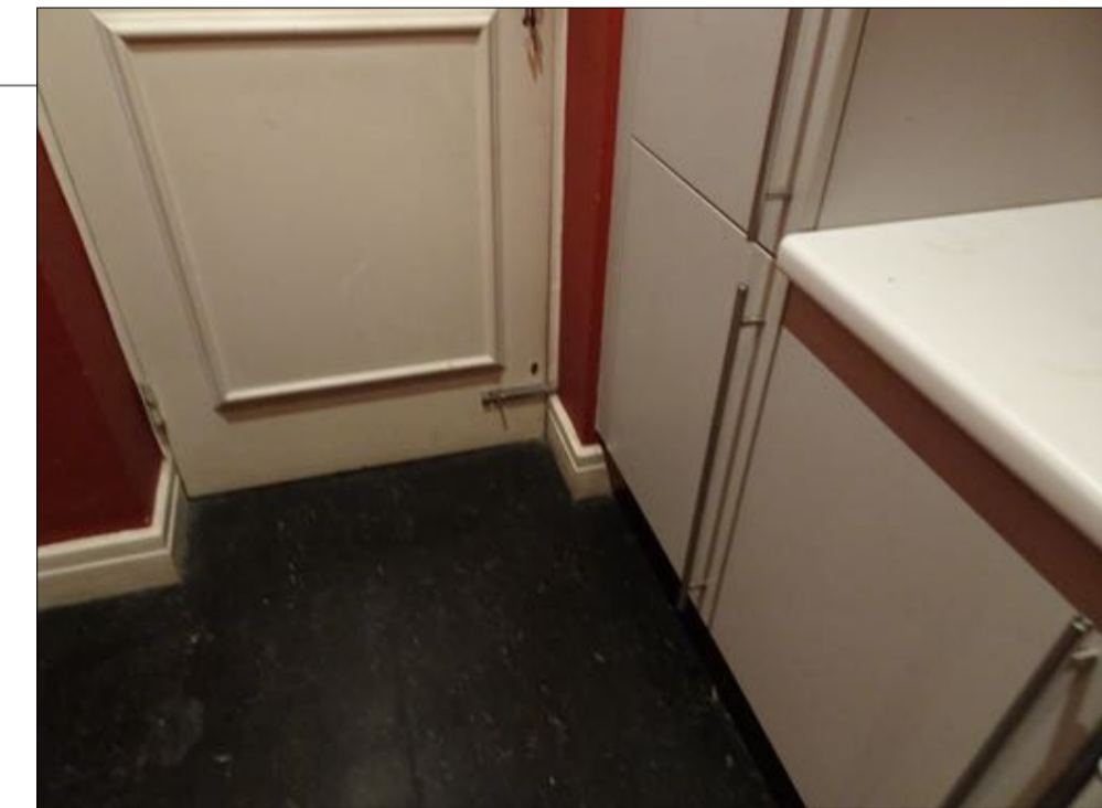
laundry units, fixtures, fittings, skirtings and floor finishes removed
