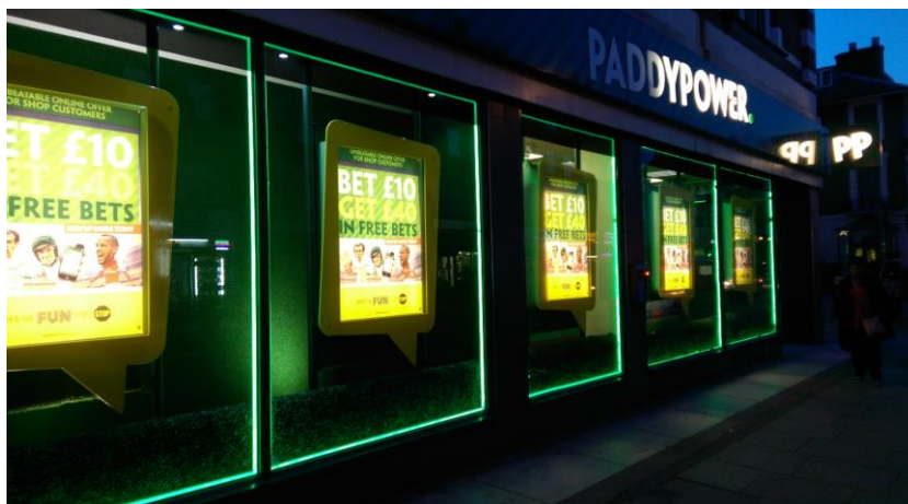
Figure 9 (left): The existing Paddy Power at 251 Kilburn High Road at night on 04/02/2016. There are no views into the premises which does not promote an active frontage or relate well to the streetscene.
