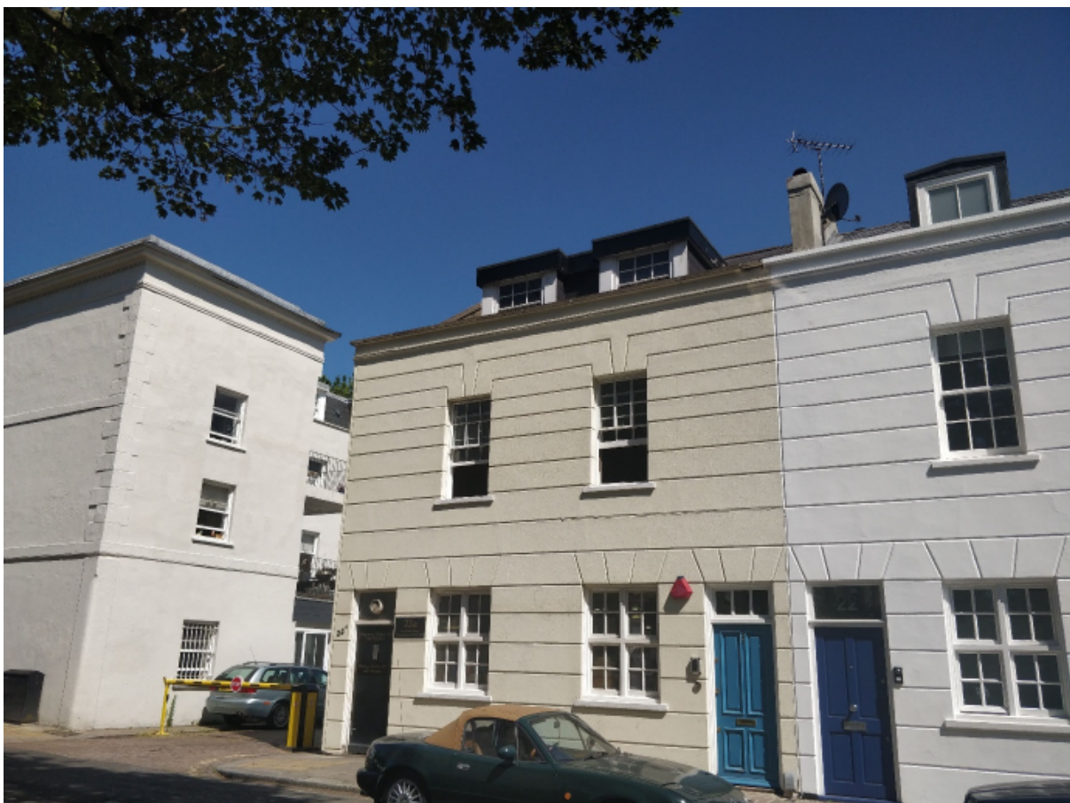
2) Front elevation of site
