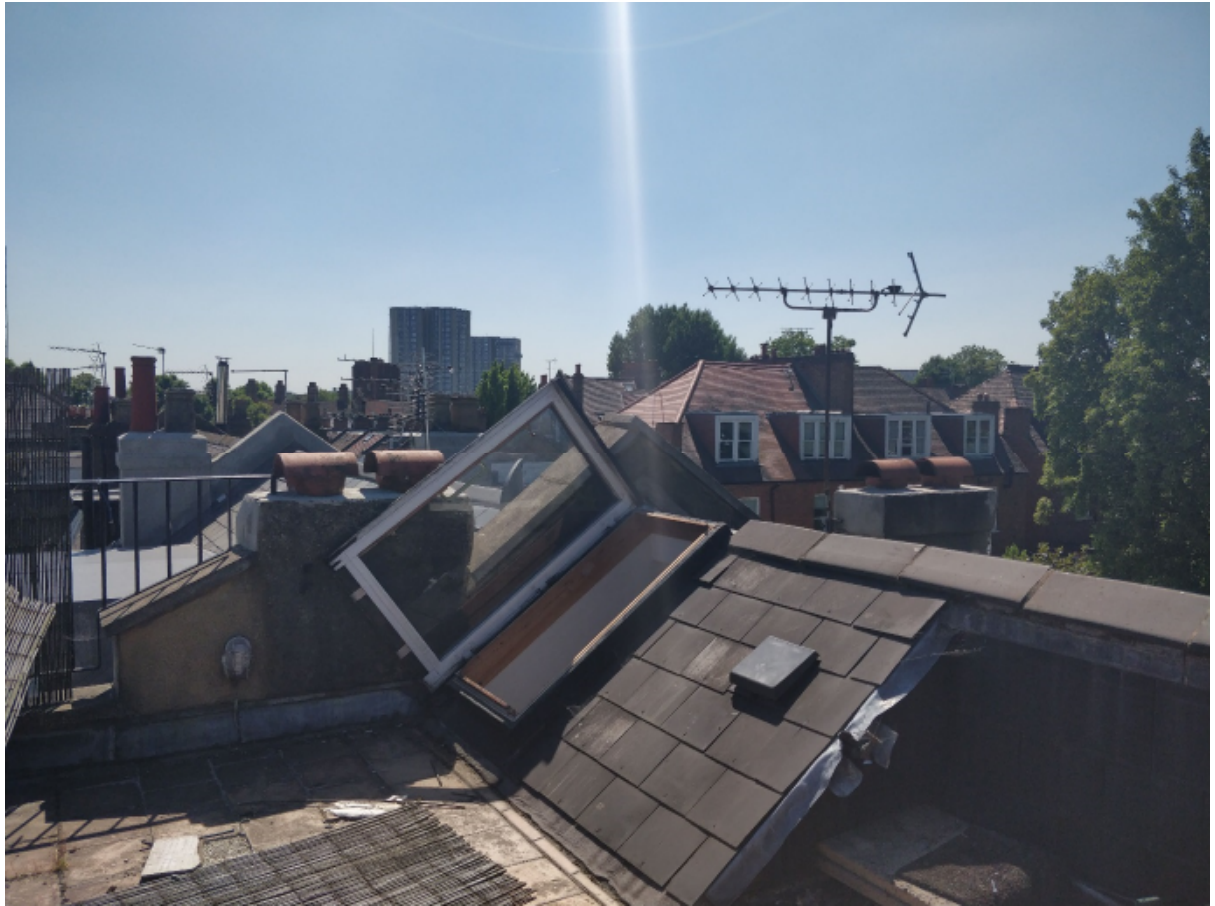
3) Existing roof access
