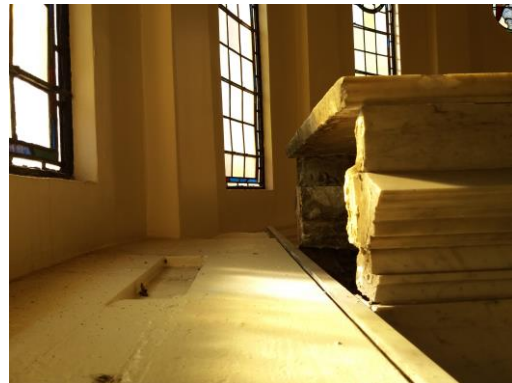
Figure 4: The rear of the altar which is clearly unresolved with the adjacent structure.
