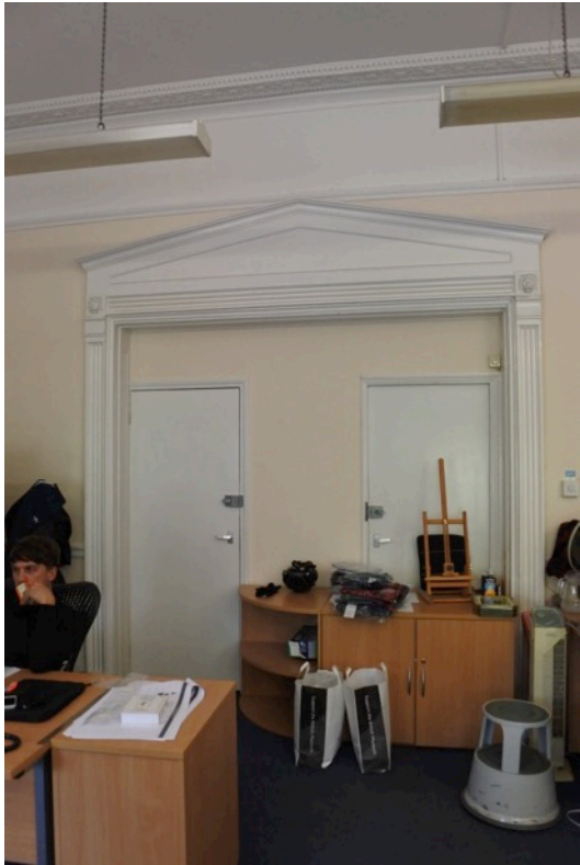
Top: Boxing to existing fireplace in First Floor. Discreet opening up works to determine if original features remain behind boxing. Mantelpiece to be revealed, repaired and redecorated if existing. Left: Modern partition infill within decorative opening to be removed to reveal open plan form. Skirting and decorative features to be repaired and reinstated. Right: Door leaves and ironmongery appear to have been altered over time. New design scheme for doors and ironmongery to comply with fire regulations and improve the look and feel.
