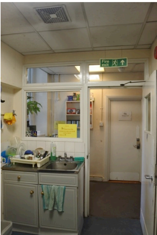
Above: Main office in Basement. Suspended tiled ceiling to be replaced with MF plasterboard MF painted ceiling with integrated lighting, heating, cooling and ventilation systems. Left: Existing WC cubicles obstructing the window to be removed. Repairs to surfaces affected by damp. Proposed improved WC layout and finishes. Georgian wire glass to be replaced with frosted. Right: Glazed modern partitions and kitchenette in corridor to be removed. New kitchenette with bespoke joinery to be provided to comply with fire regulations.
