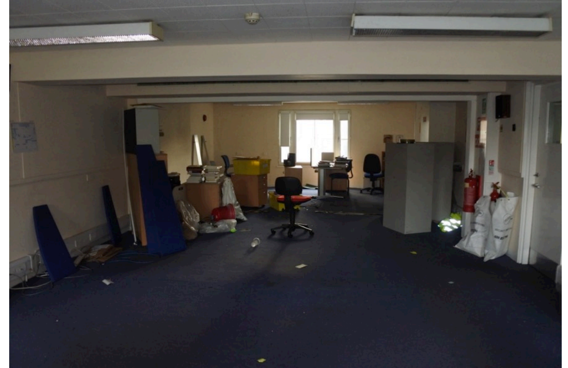
Above and Below: Existing soffit mounted ceiling tiles and redundant services to be removed. Damp issues to ceiling to be rectified. Existing soffit to be repaired and redecorated.
