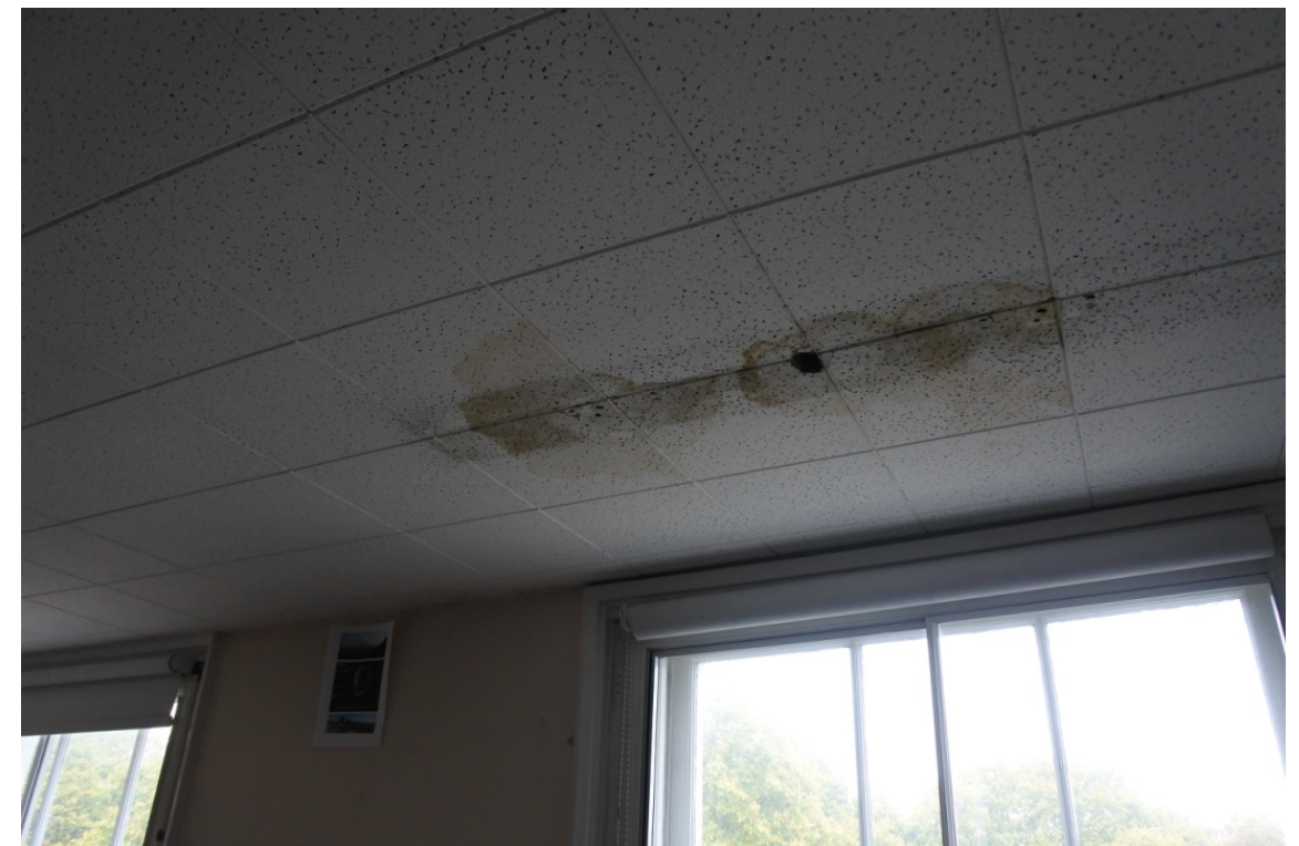
Above and Below: Existing soffit mounted ceiling tiles and redundant services to be removed. Damp issues to ceiling to be rectified. Existing soffit to be repaired and redecorated.
