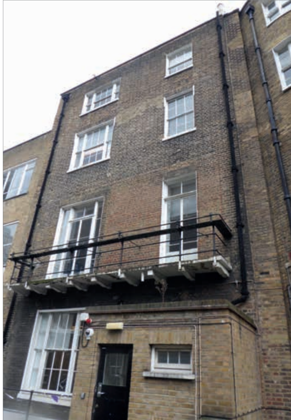
Figure 6.4 Photograph of the rear elevation of number 43
