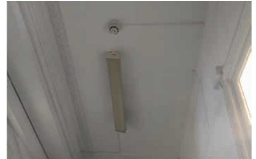
Figure 6.20 Former fire partition roller shutter at no. 43
