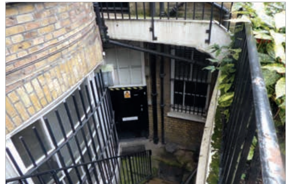
Figure 6.6 Rear access to the basement of no. 43
