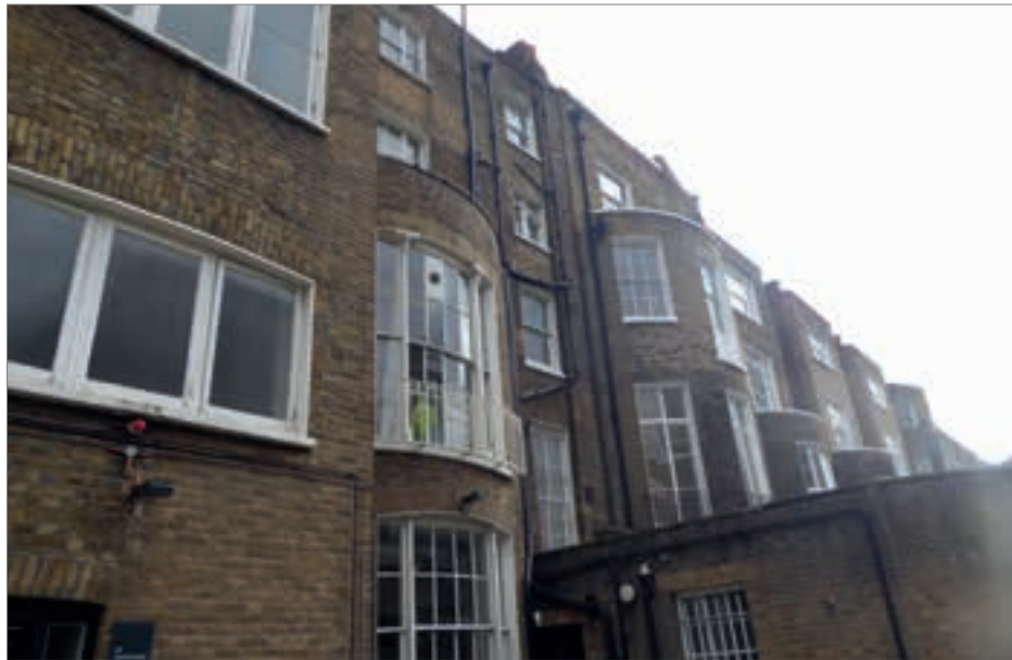
Figure 6.2 Photograph of the rear elevation of number 42
