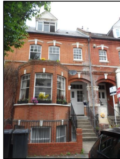
Figure 2 – Front Elevation of No. 15
