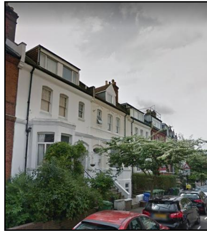
Figure 6 – Properties on opposite side of road
