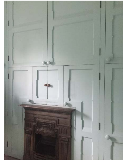
Fire surround applied to the face
