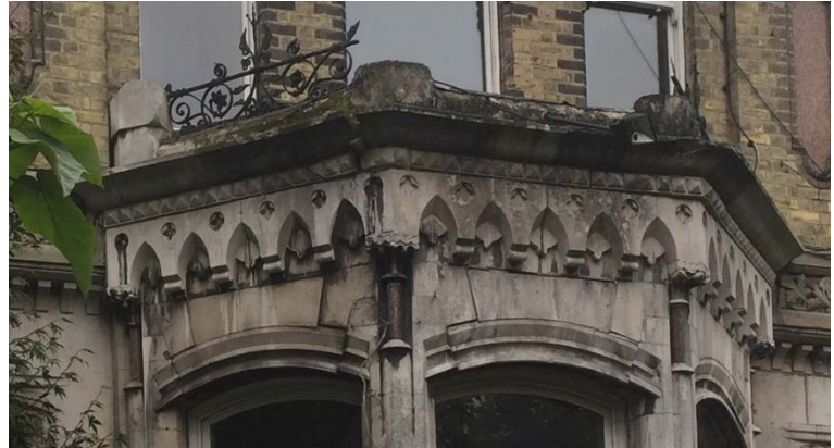
9.1 Original 1868 etching 9.2 Showing partial balustrade and deformation of stonework.
