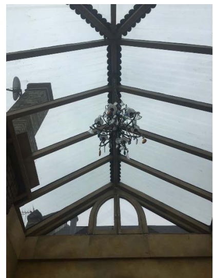
14.3 Modern glazed roof behind existing chimney
