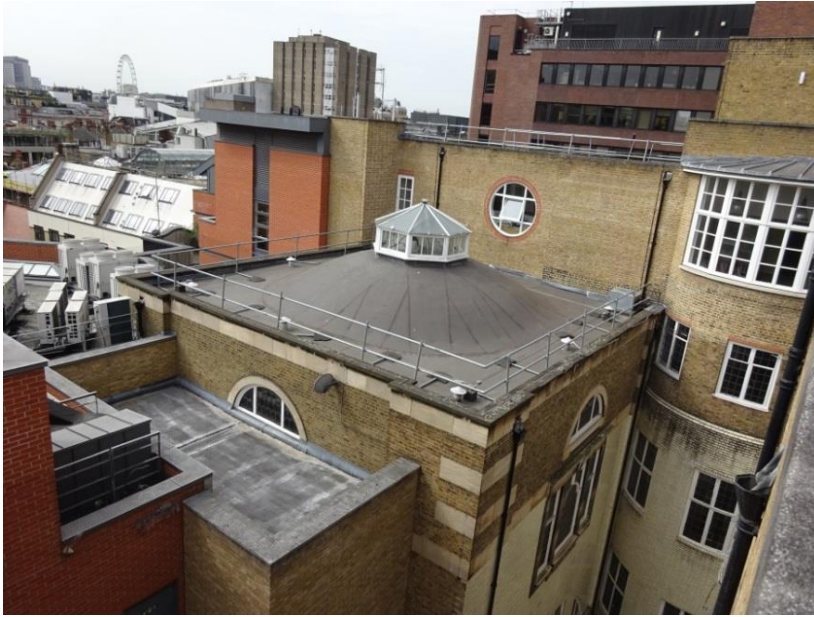
Figure 20: View south from roof of site (eastern wing)
