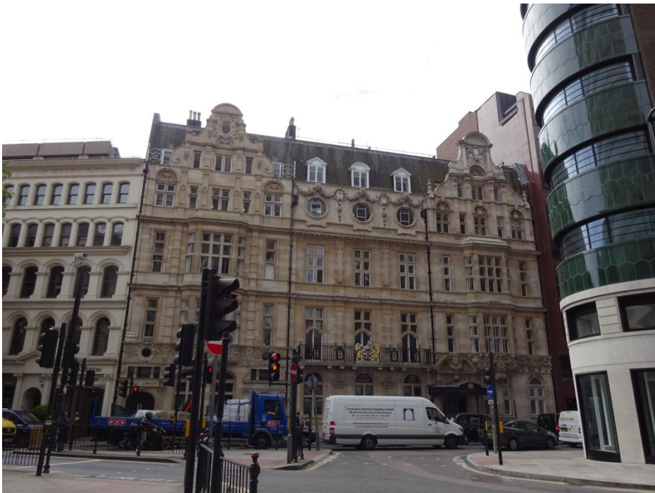
Figure 14: View of Holborn Town Hall from junction opposite
