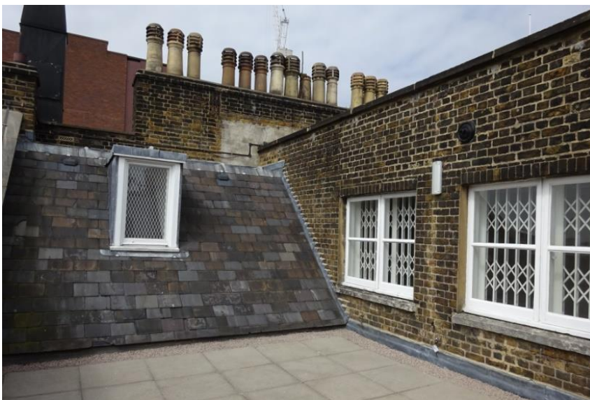
Figure 26: Boxed out area to office 5B with slate roof
