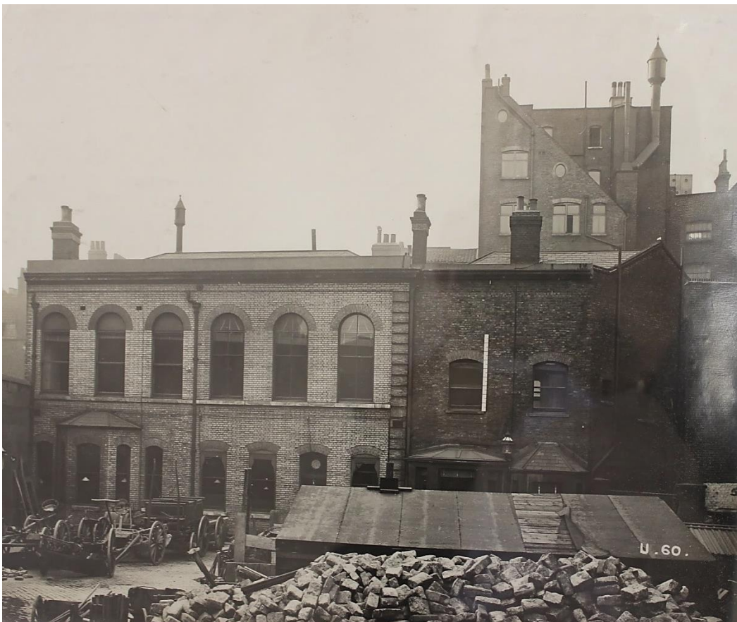
Figure 7: Rear view of Holborn Library and Town Hall
