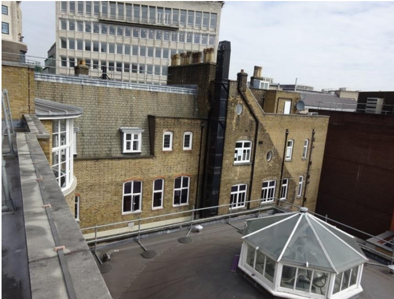
Figure 18: View north from roof of site
