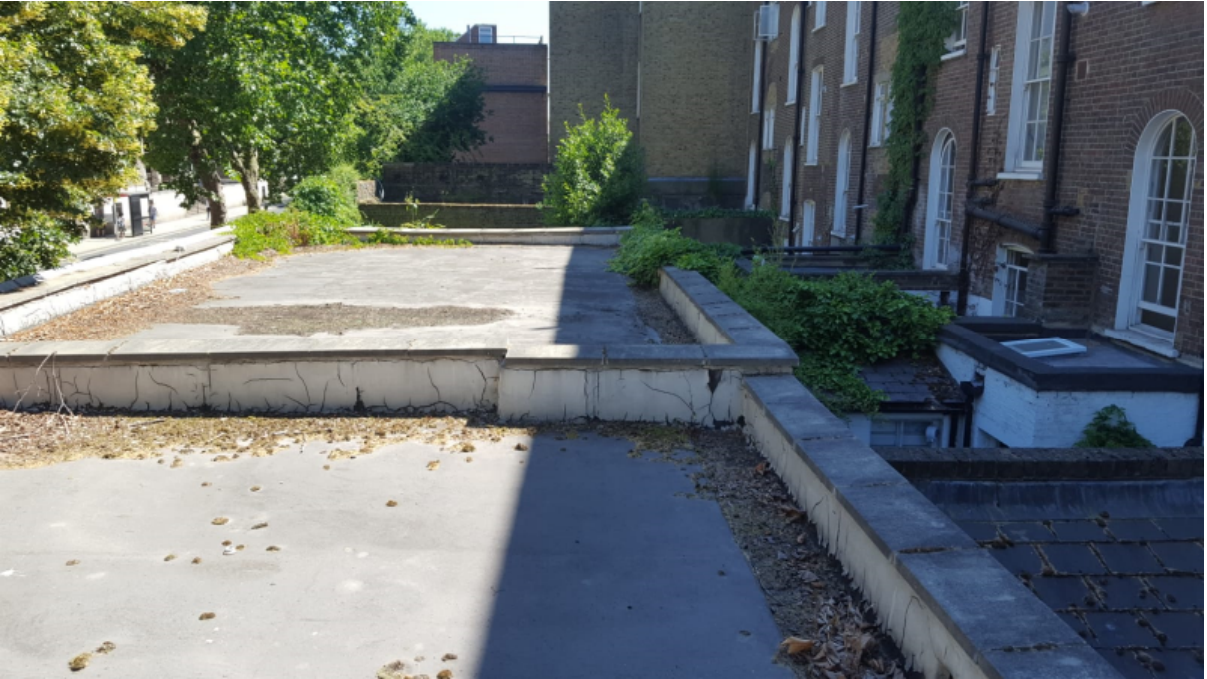
3. Rooftop looking south
