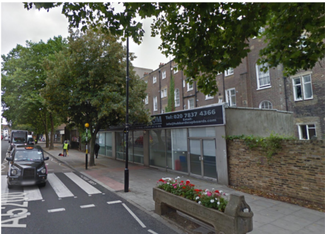
2. Front looking south
