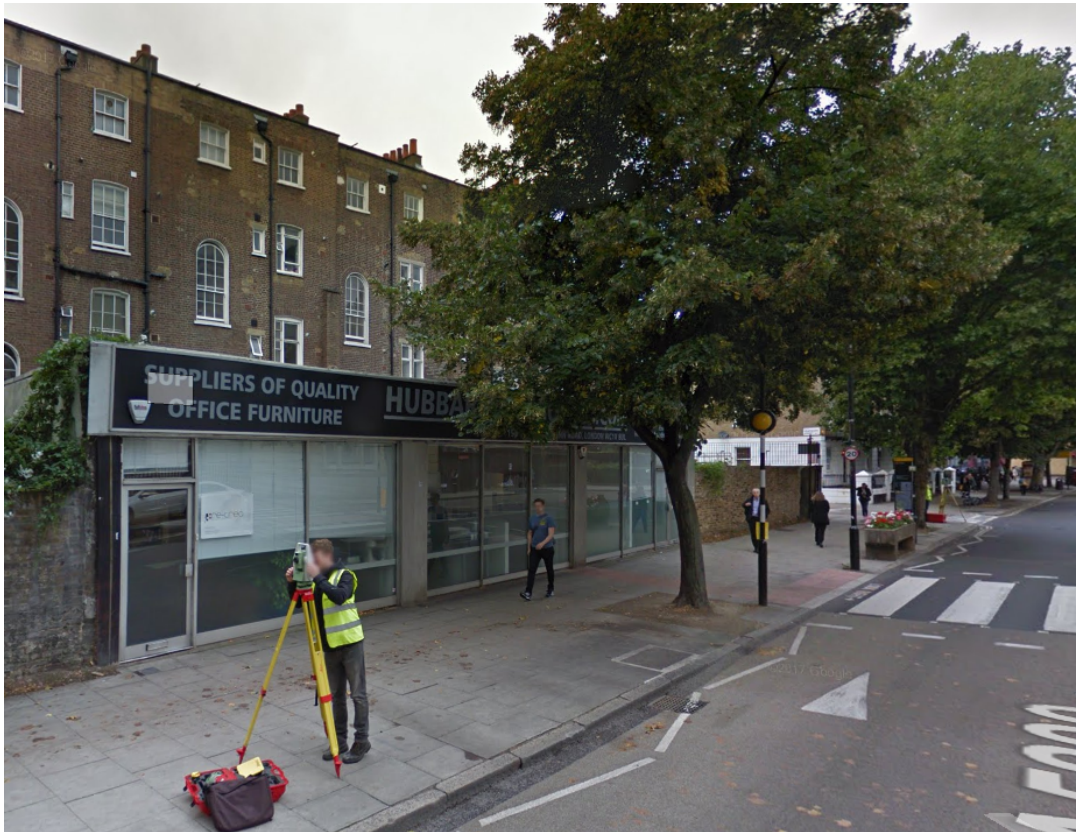
1. Front looking north
