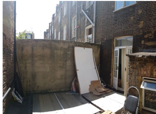
Rear of site, looking towards party wall against No.200
