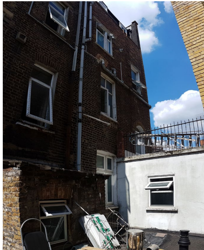
Rear of site looking towards adjacent site extension (No. 204)
