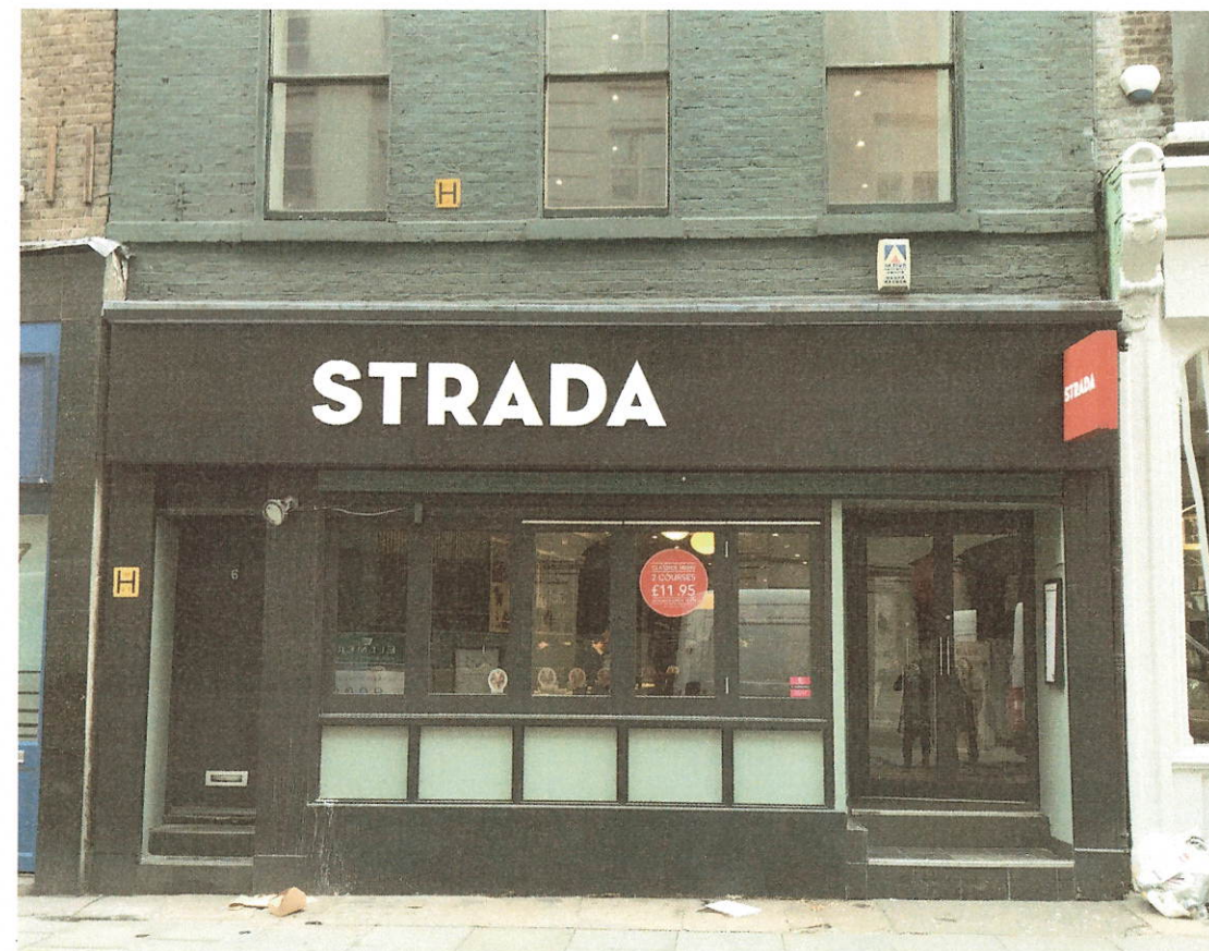
Existing shopfront reference
