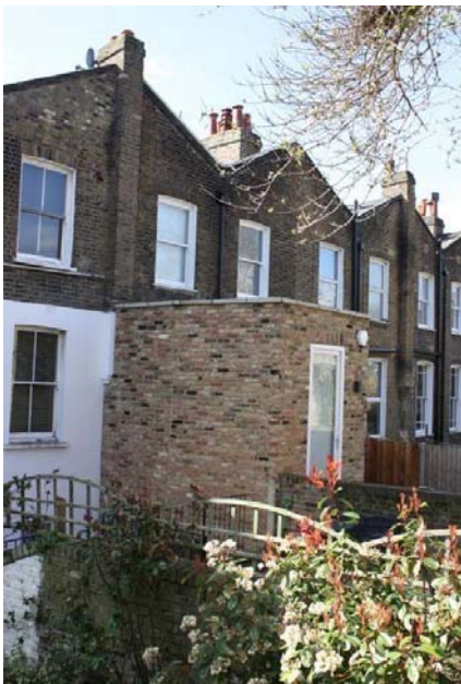
Left: Photo of extension to no. 48 from garden of no. 44
