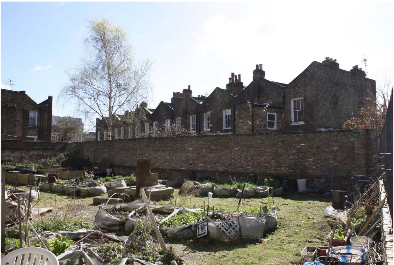
Above: rear view of Coity Rd Terrace from Bassett St – note only the three storey extension to no. 56 is visible. All other extensions (no. 44, 48 & 54) are not.
