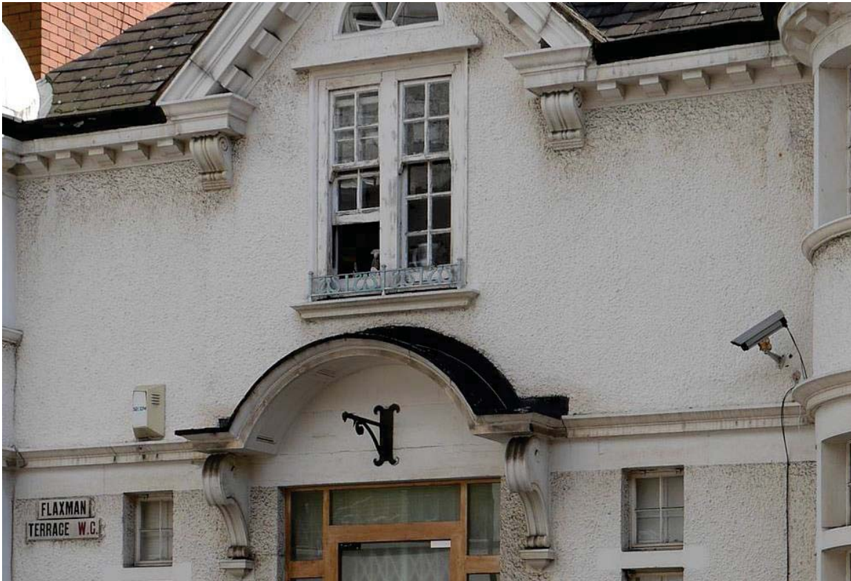
Fig 51 The original bracket for a lantern above door D1 in 2013
