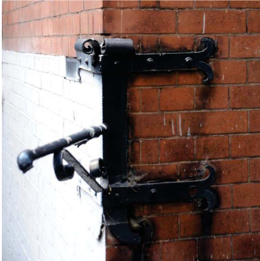
Fig 17 The gas light bracket on the north-east corner of The Lodge
