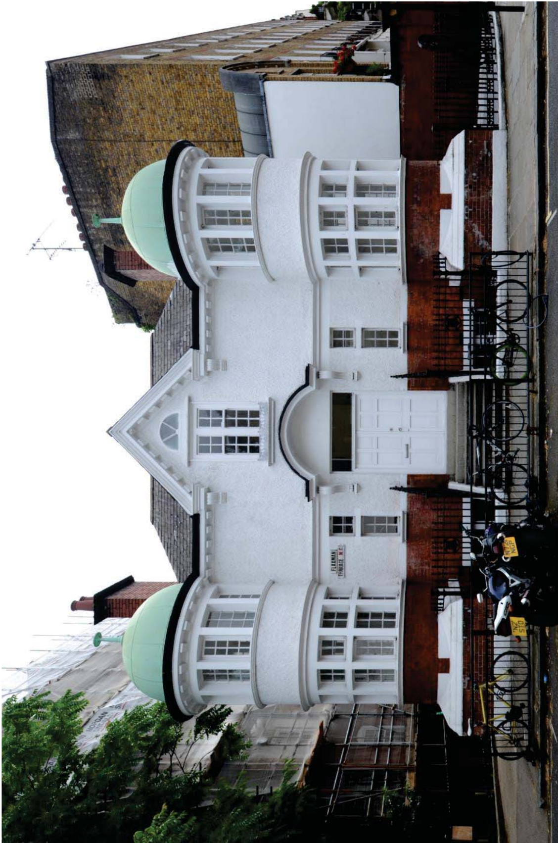
Fig 3 The Lodge from the west
