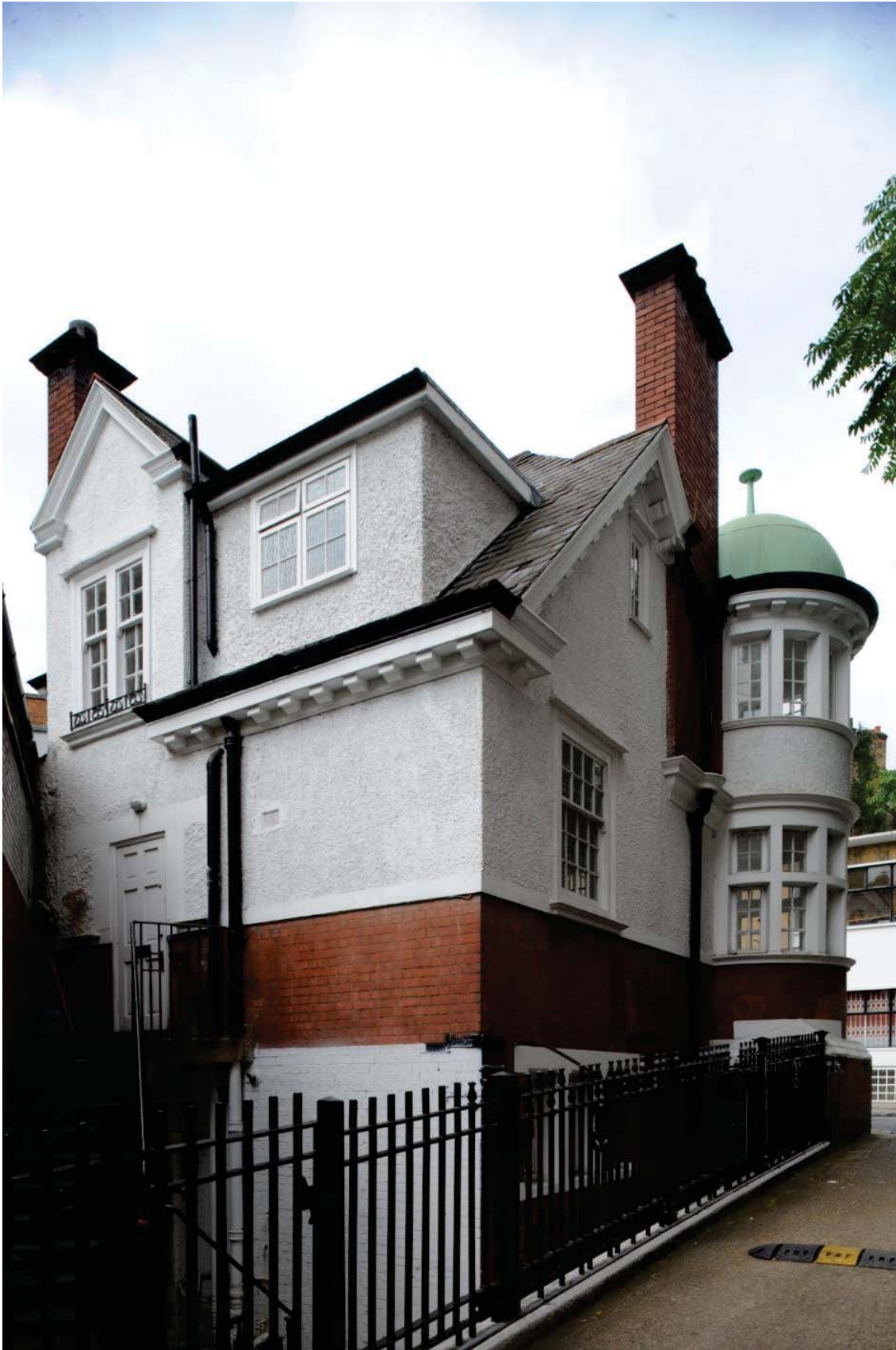
Fig 4 The Lodge from the north-east
