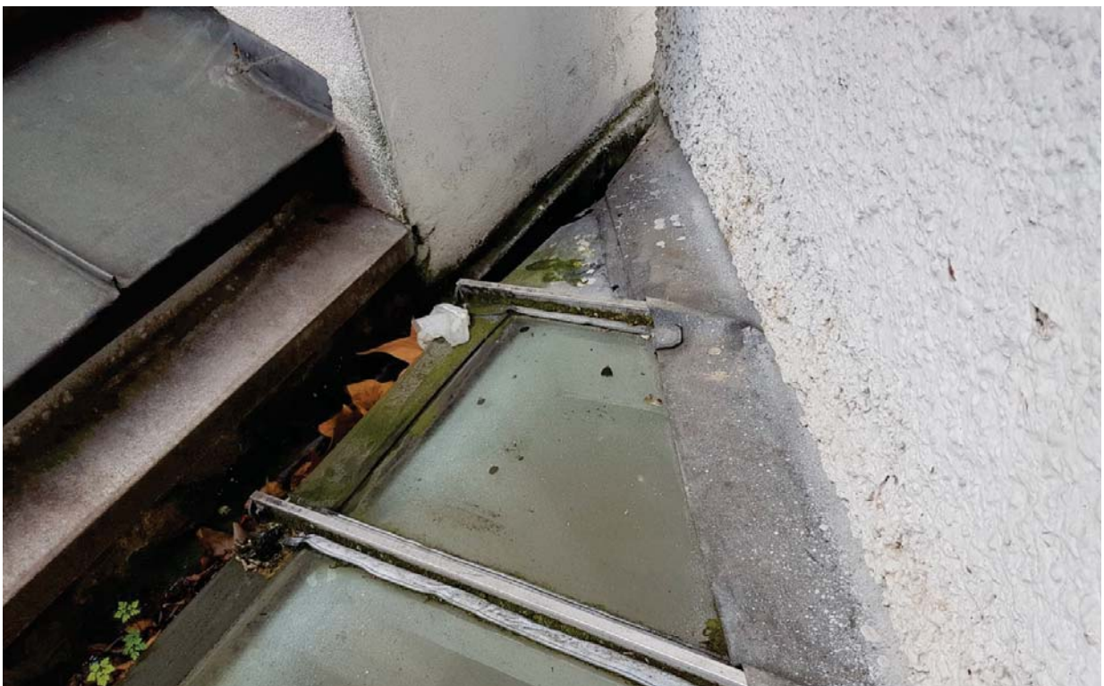
Fig 52 The north end of the glazed roof
