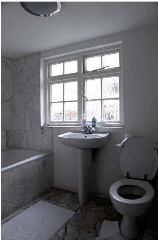
Fig 26 The bathroom and toilet on the first floor
