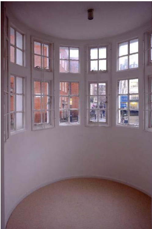
Fig 21 The south-west tower on the ground floor
