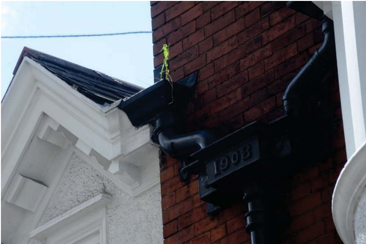
Fig 6 The rainwater hopper dated 1908 on the north elevation
