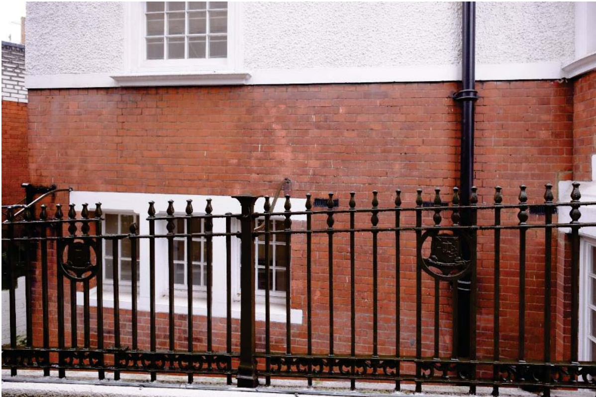
Fig 48 The original iron railings to the north area
