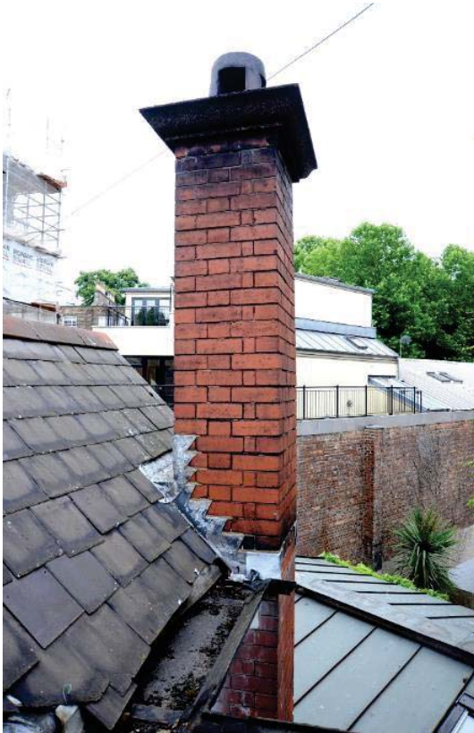
Fig 12 The east chimney stack
