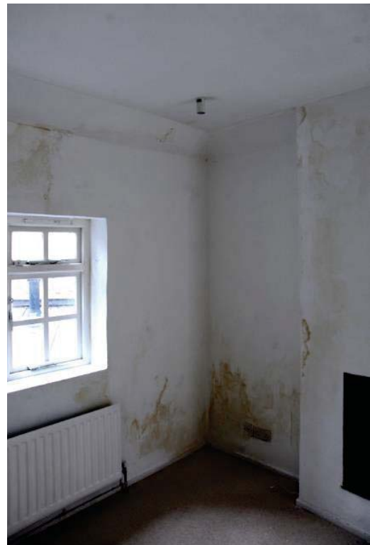
Fig 27 The south-east corner of the south room on the first floor
