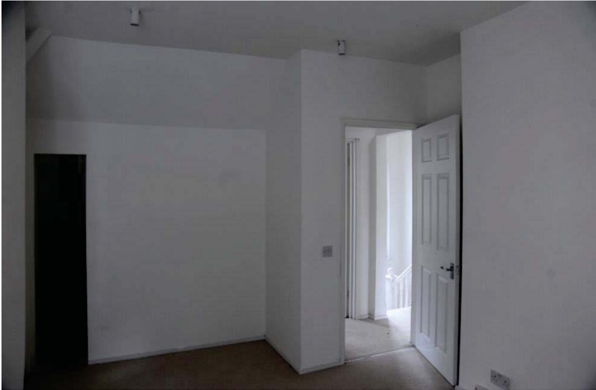
Fig 25 The east wall of the north room at first floor level
