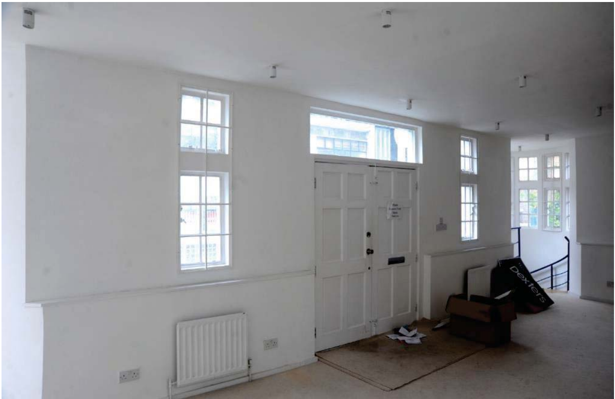
Fig 34 The west wall of the ground floor space
