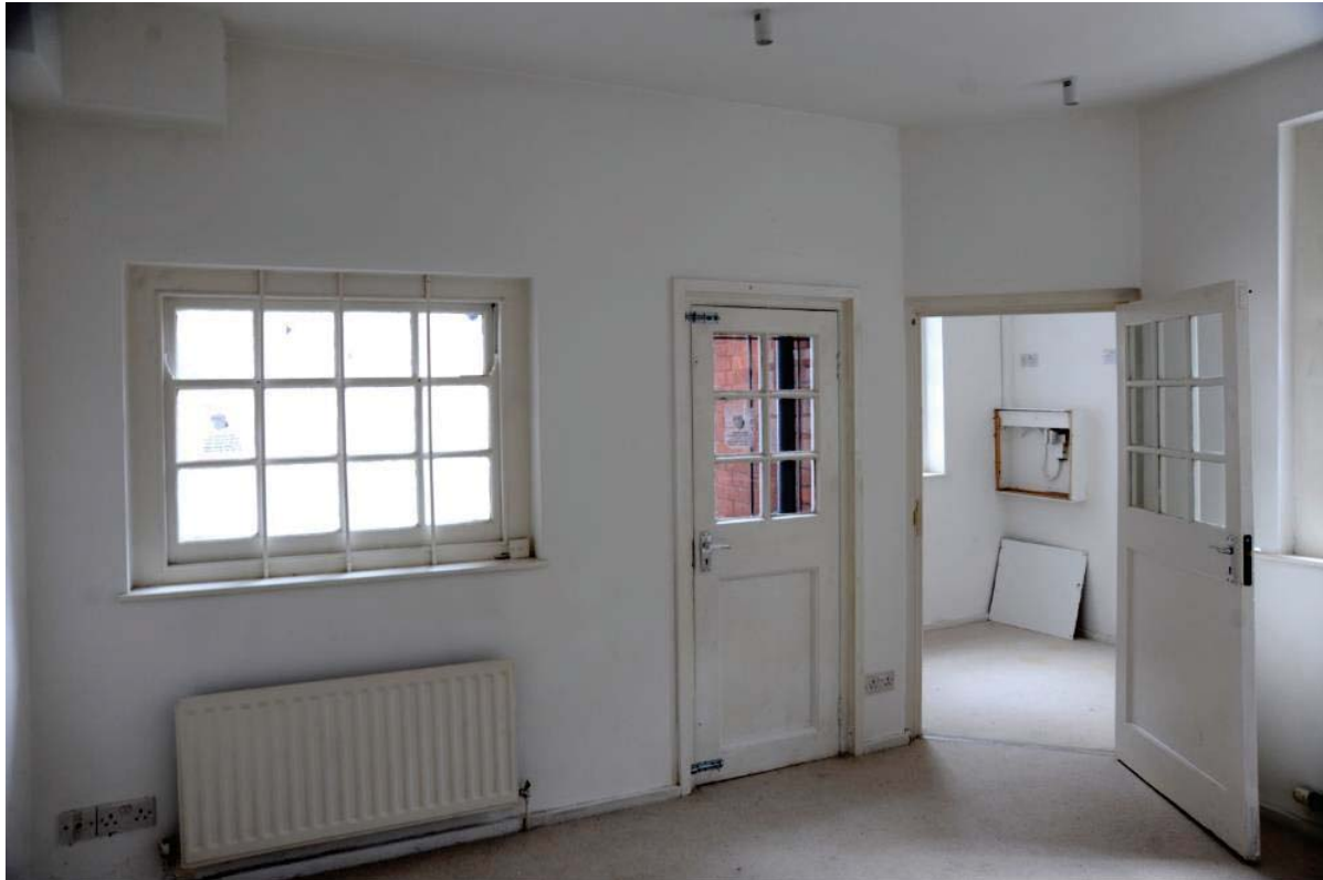
Fig 39 The south wall and door to the south-west tower at basement level
