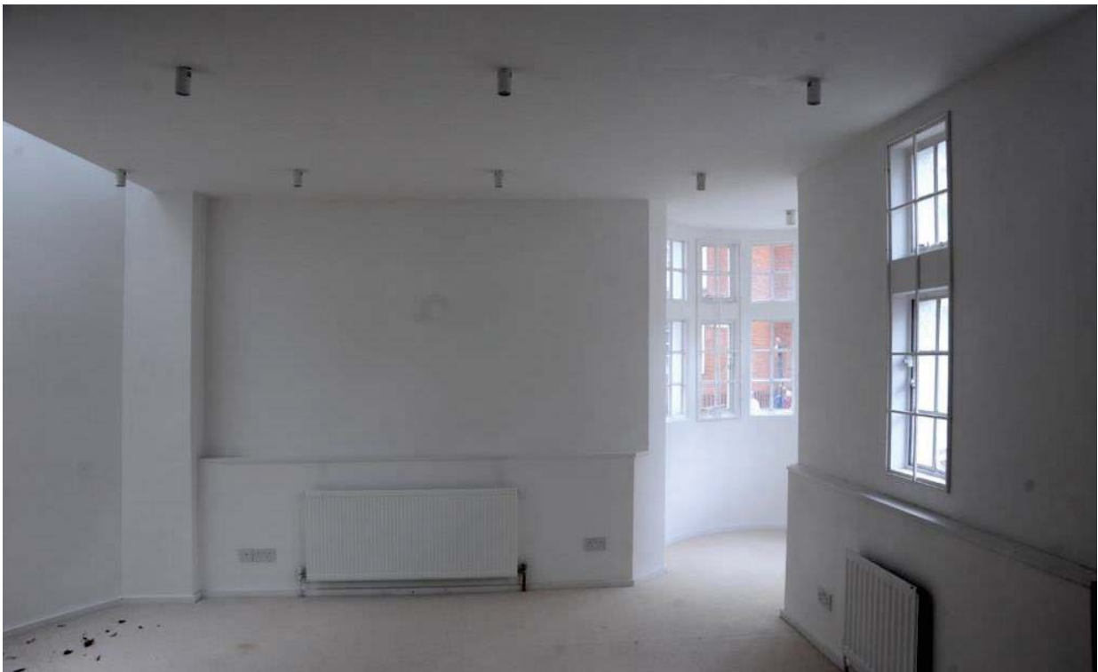
Fig 32 The ground floor space looking south
