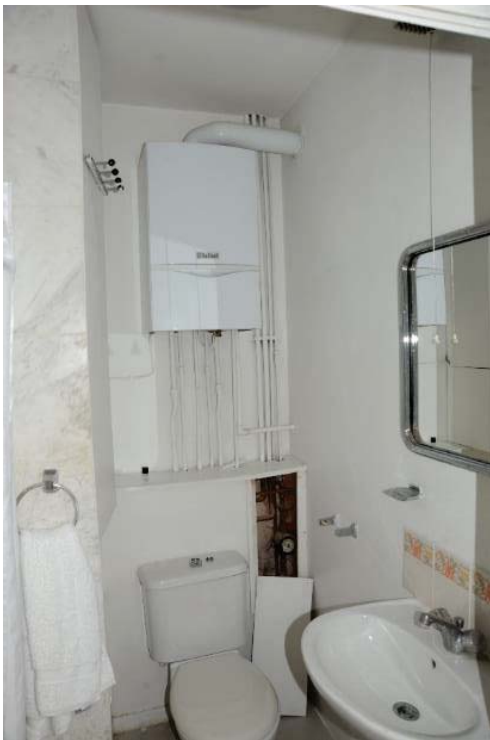
Fig 41 The shower room and toilet in the basement
