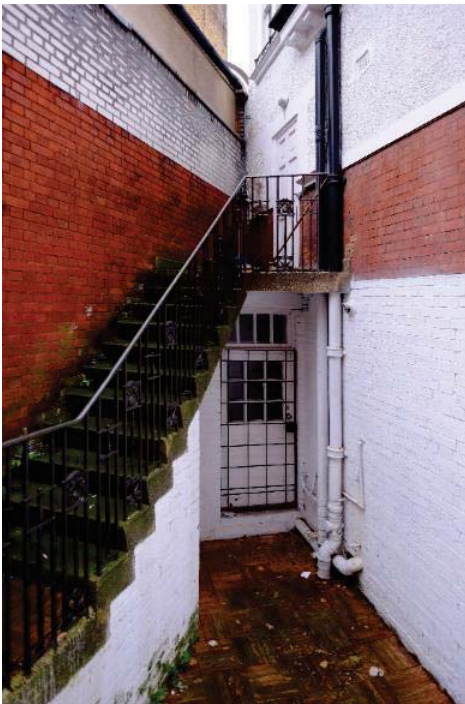
Fig 18 The rear doors and external stair in the east area
