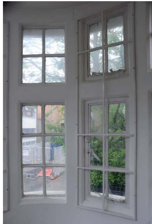
Fig 22 Ground floor windows in the north-west tower
