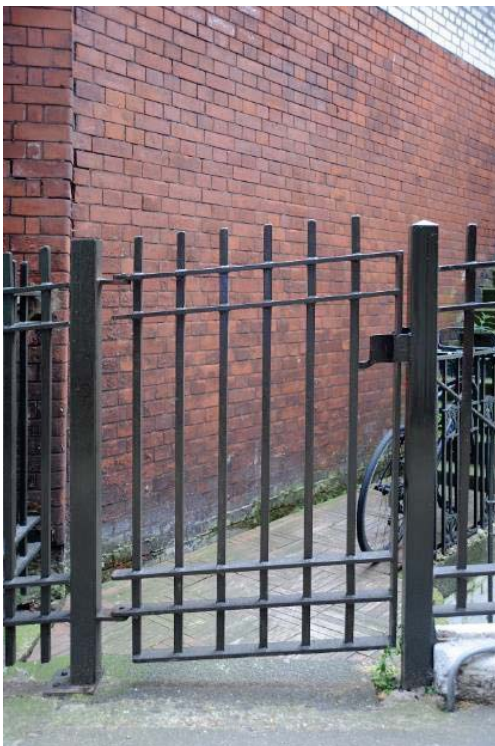
Fig 49 The modern rear gate giving access to the east area
