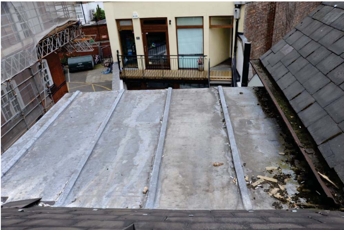
Fig 7 The lead roof over the rear dormer
