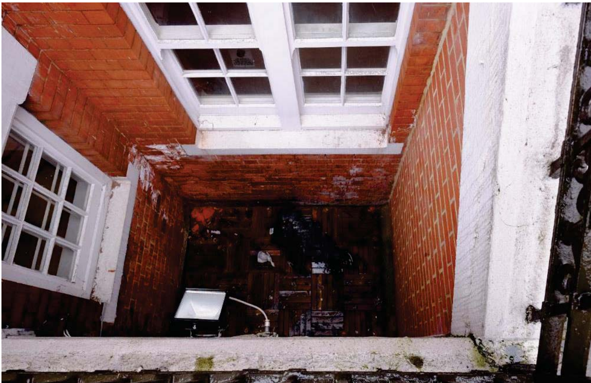
Fig 14 The north lightwell on the west side of The Lodge
