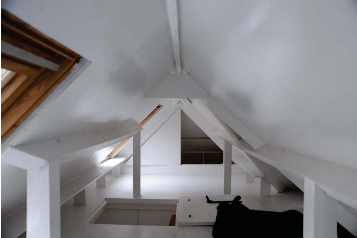
Fig 23 The attic looking south
