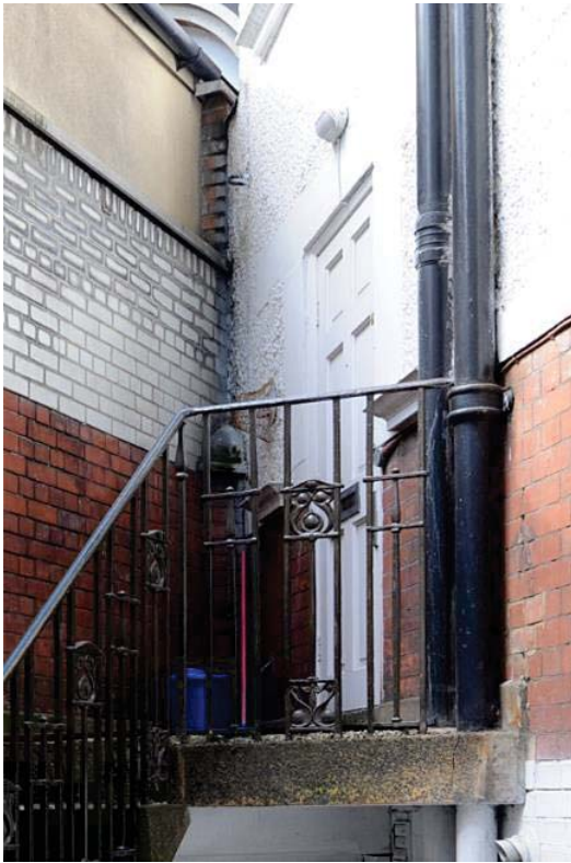
Fig 35 The landing outside door D2
