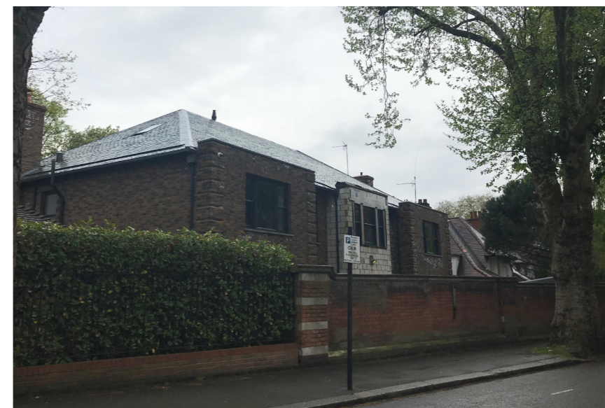
Image of front elevation as currently constructed and proposed in this application (natural stone to be added to front central bay)
