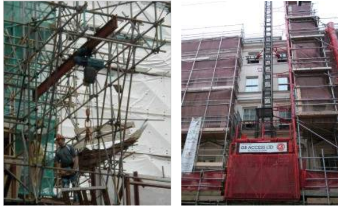
Figure 8: Proposed lifting beam and goods hoist
