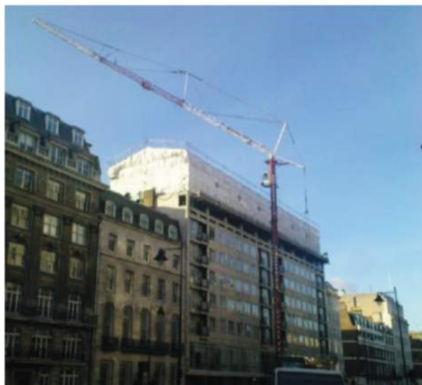
Figure 10: Example BHCLtd roof extension scaffold at Ambika House
