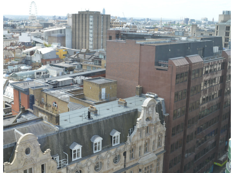
High Level View Looking South 'As Existing'
