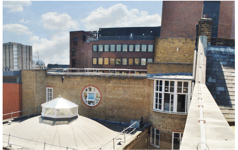
View from 5th Floor Looking West 'As Existing'
