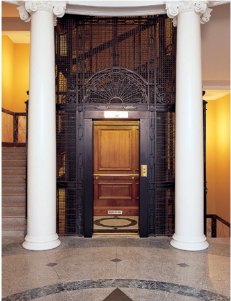
Wrought iron lift enclosure at ground floor level
