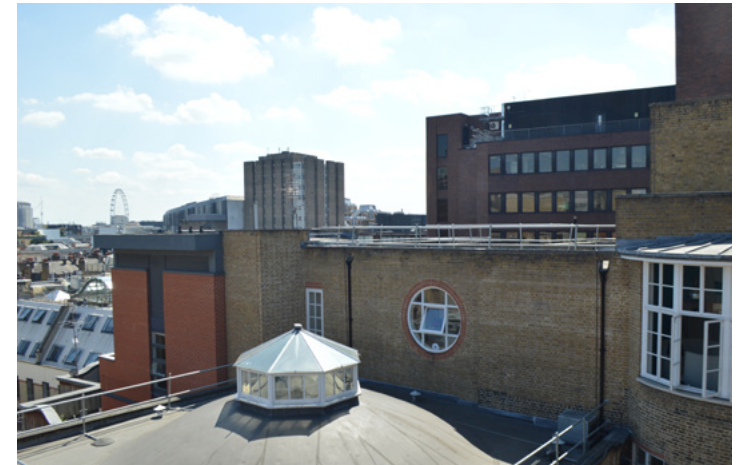
Photograph from the fifth floor East terrace showing the proposed location for the extension.
