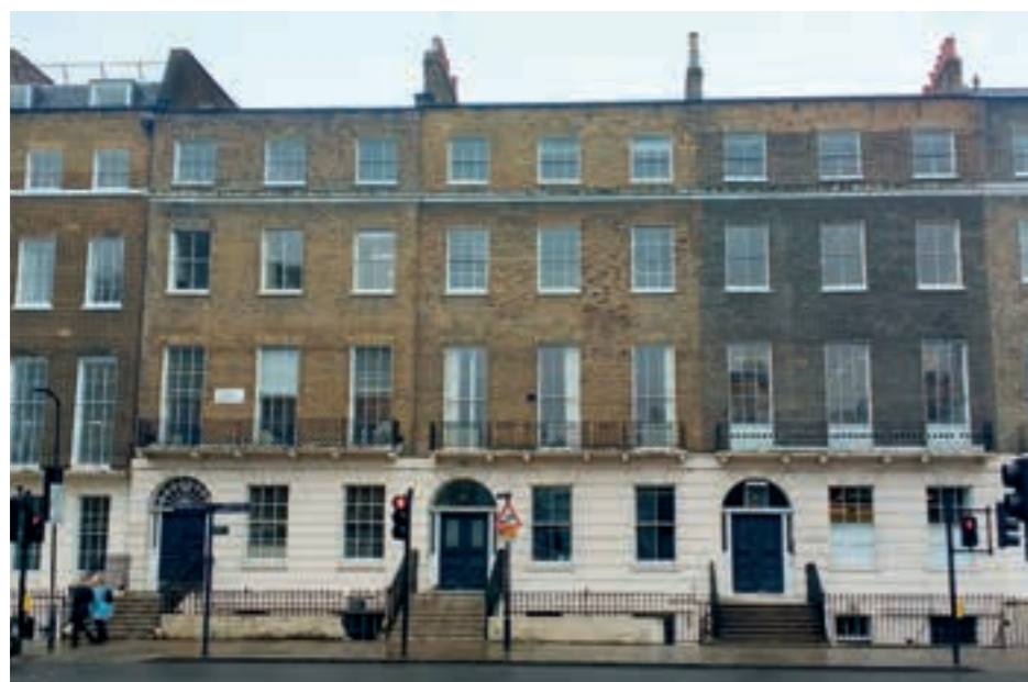
Figure 1.2 Photograph of the principal elevations of the properties to 41-43 Russell Square to the Square
