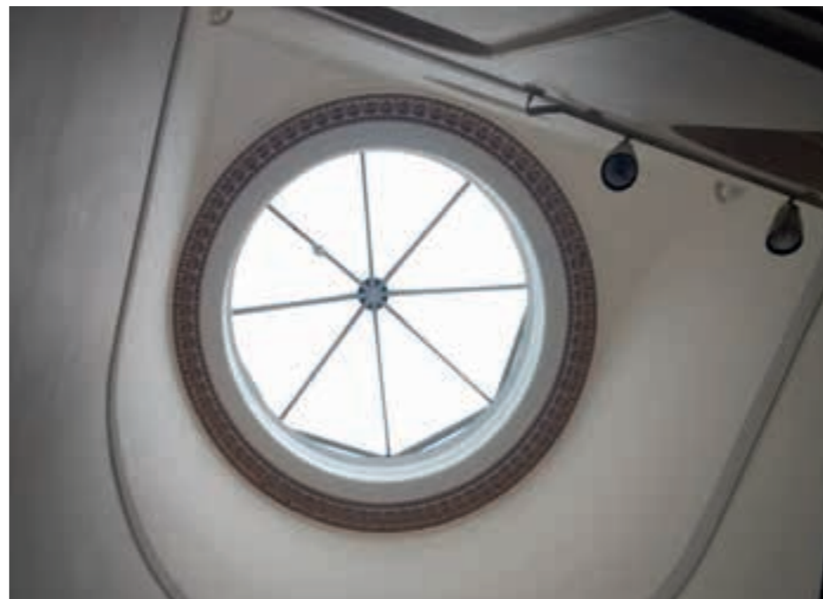
Figure 4.9 The lantern at no. 41
