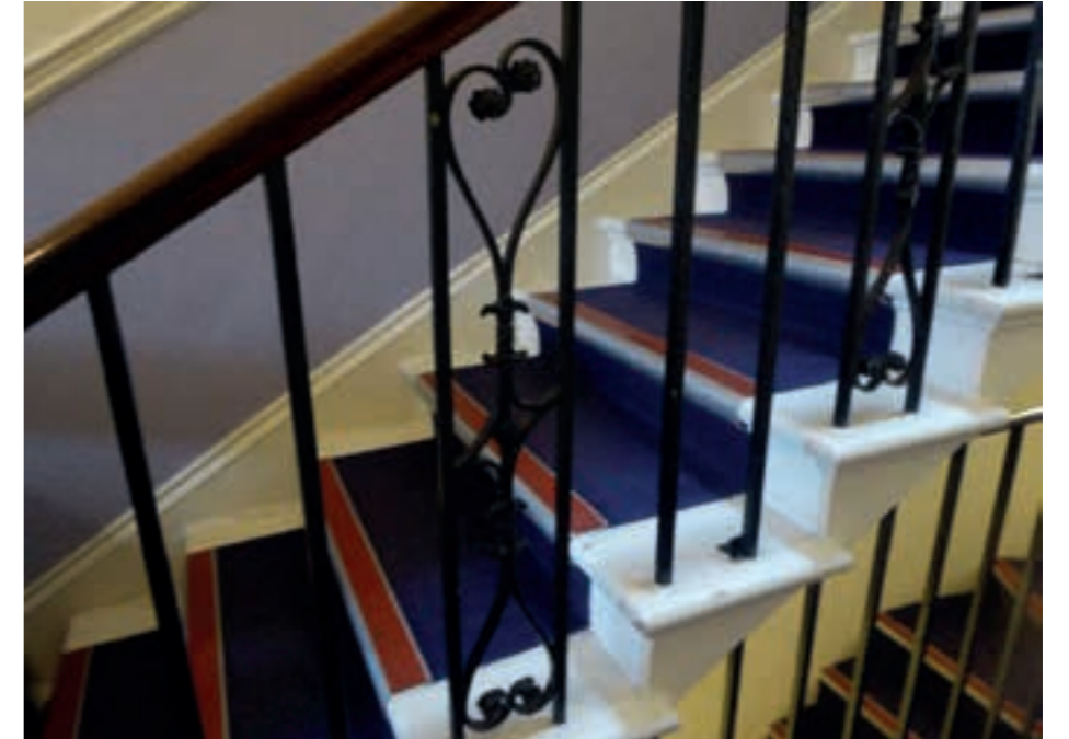
Figure 4.4 Detail of wrought iron balusters
