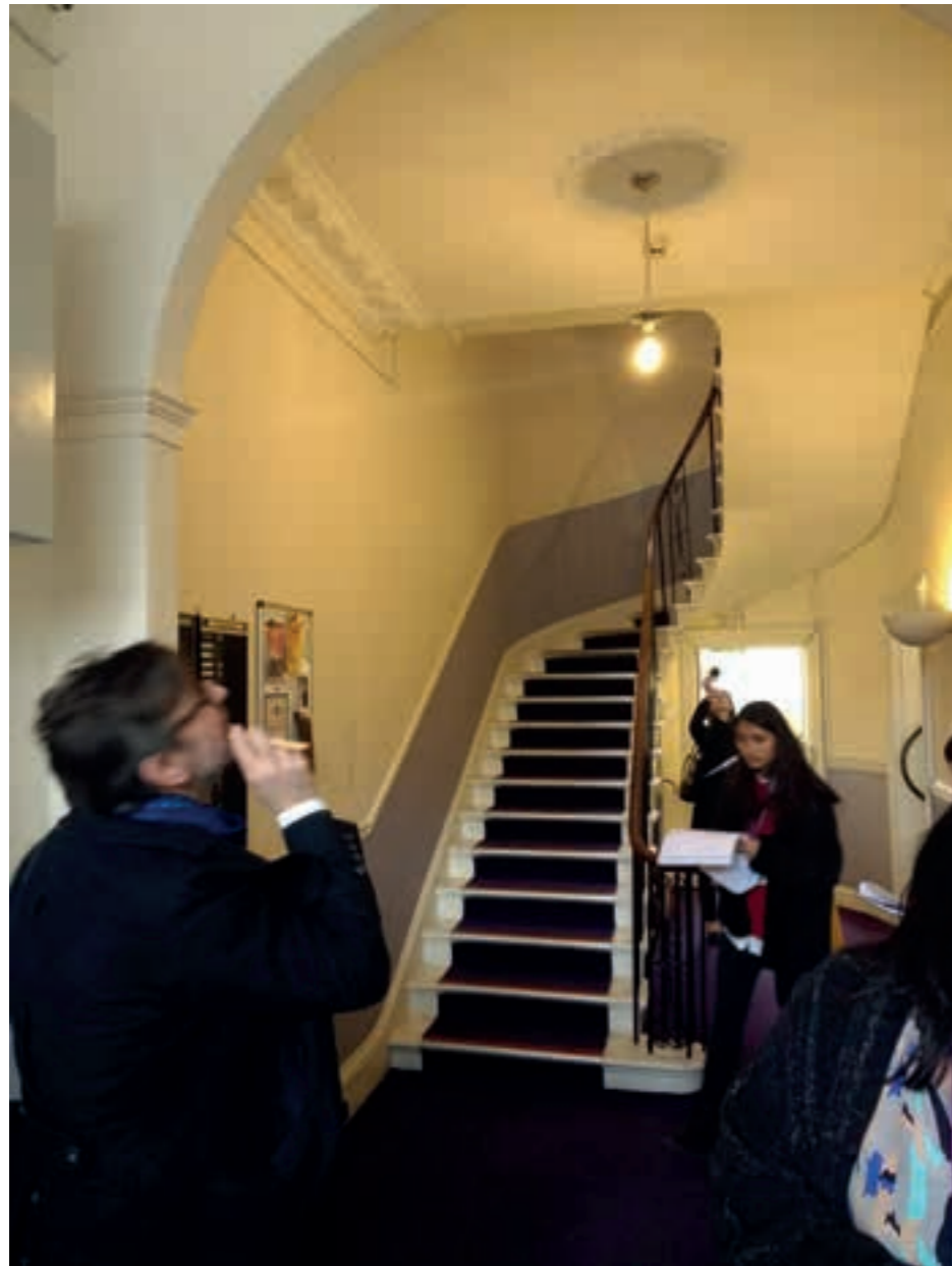
Figure 4.2 Main hallway and view of the cantilevered stair at no. 41
