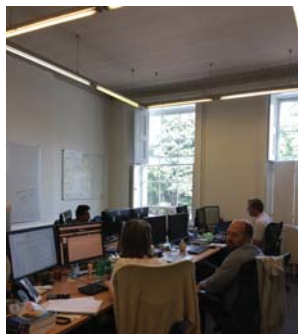
Above : Condition of Principal Rooms at 41 Russell Square
