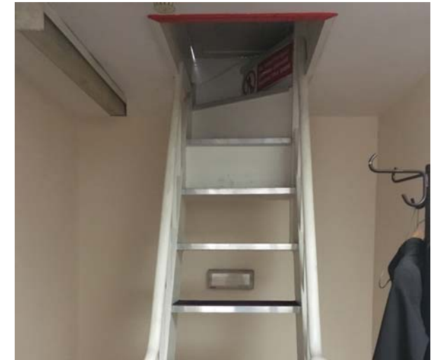
Staircase to access roof.
