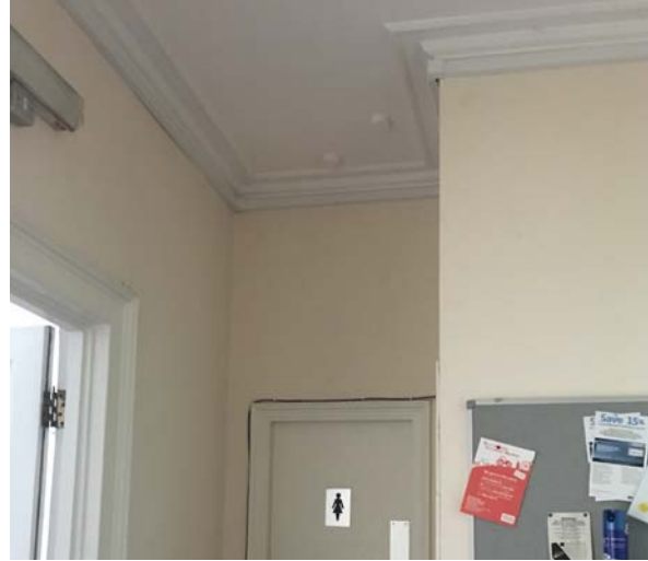
Looking at WC Doors and corridor
