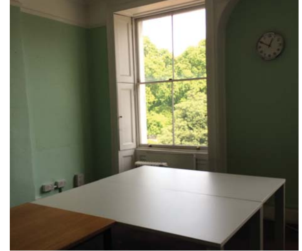
Looking at existing windows and shutters in the front office
