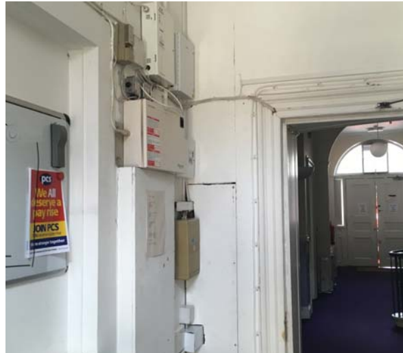
Surface mounted conduits and cables in kitchen.
