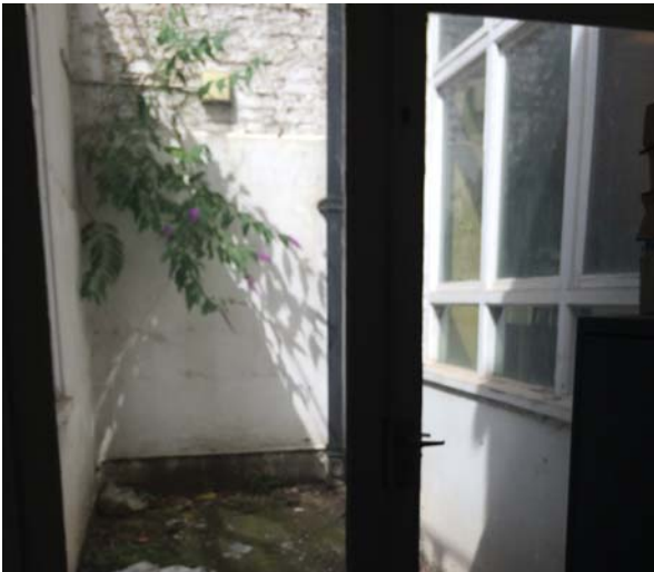
Rear external lightwell.
