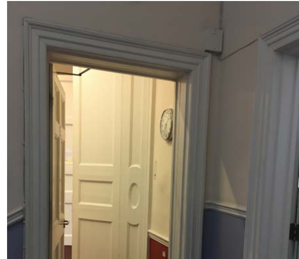
Ornate architraves with surface run cabling.
