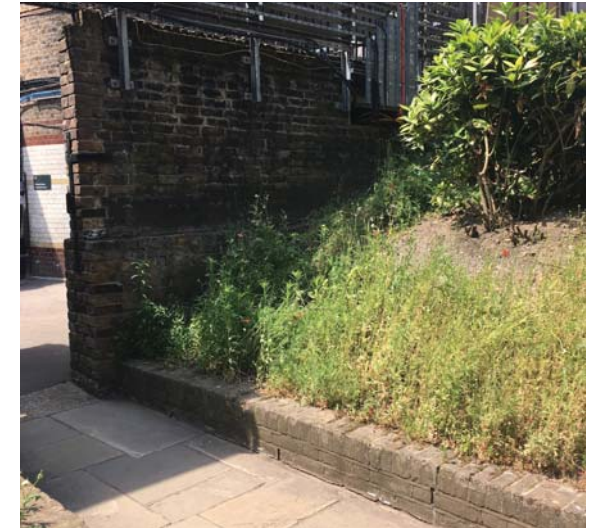
Above: Photographs showing the existing condition of the rear garden.
