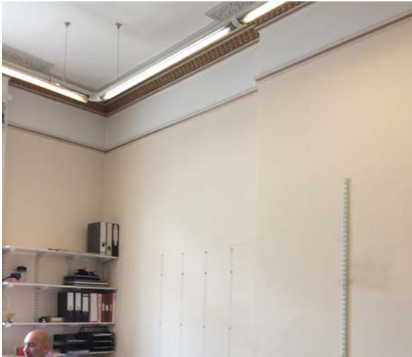
Rear office cornicing and shelving brackets.
