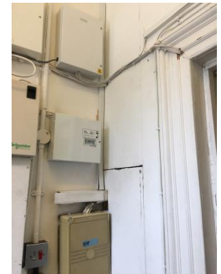
Example of existing riser and services
