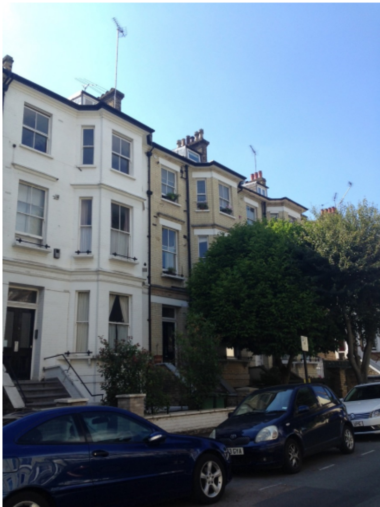
5. Front of 7 Crossfield Road
