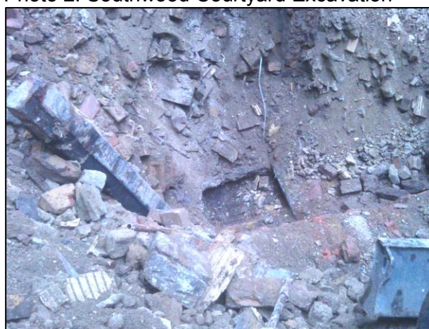
Photo 2: Southwood Courtyard Excavation
