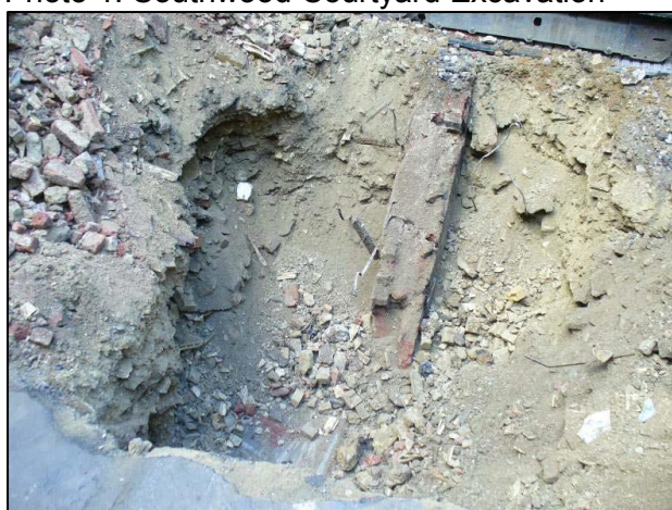
Photo 1: Southwood Courtyard Excavation
