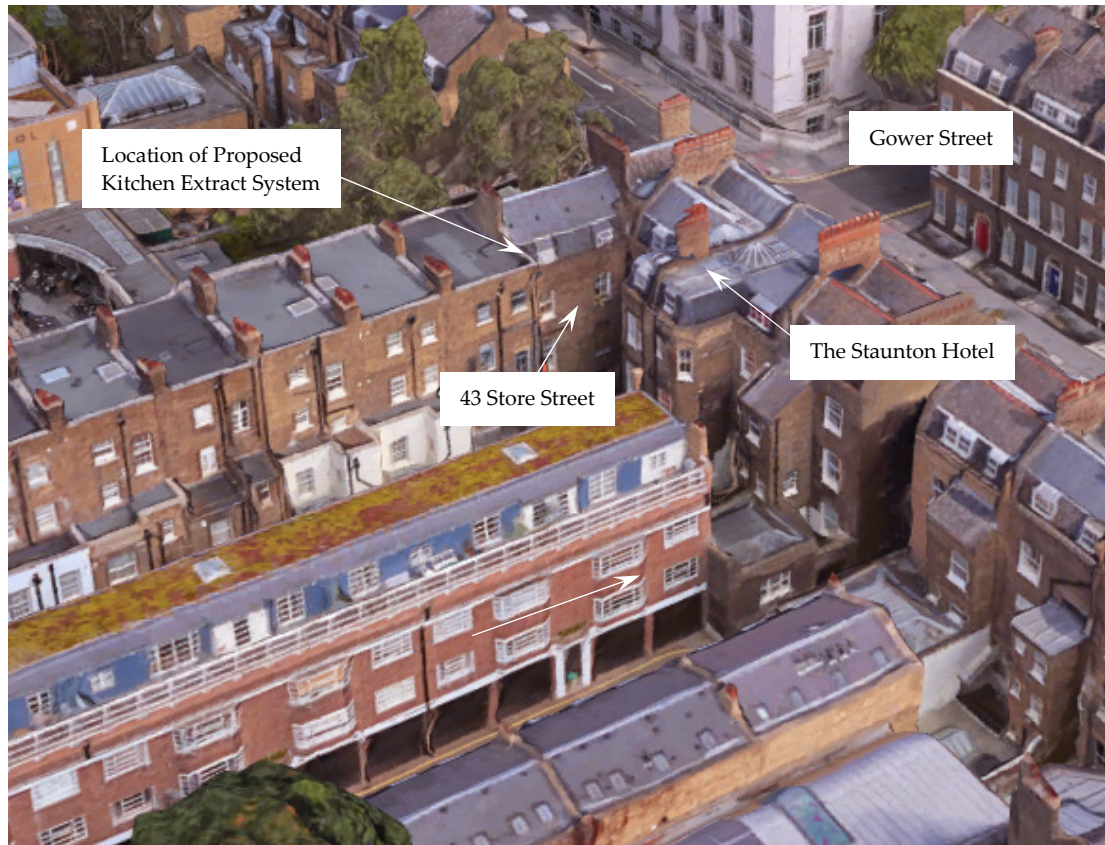
Figure 1: Site Location (© Google Maps) – 43 Store Street (from rear)
