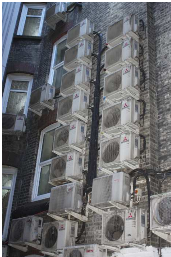
Figure 3: Existing hotel external a/c units
