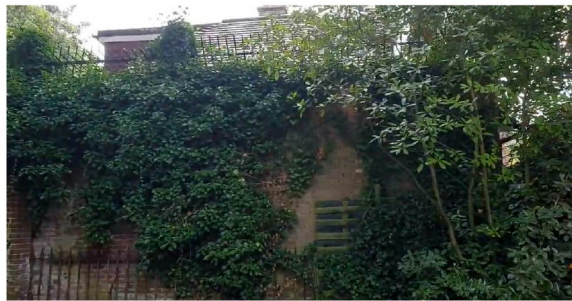
Neighbouring garage structure to the south
