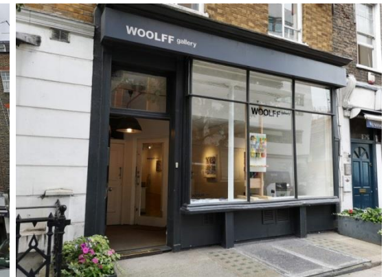
GROUND FLOOR SHOPFRONT TO GALLERY
