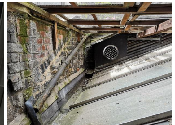
GLAZED ROOF BELOW PIGEON PROTECTION
