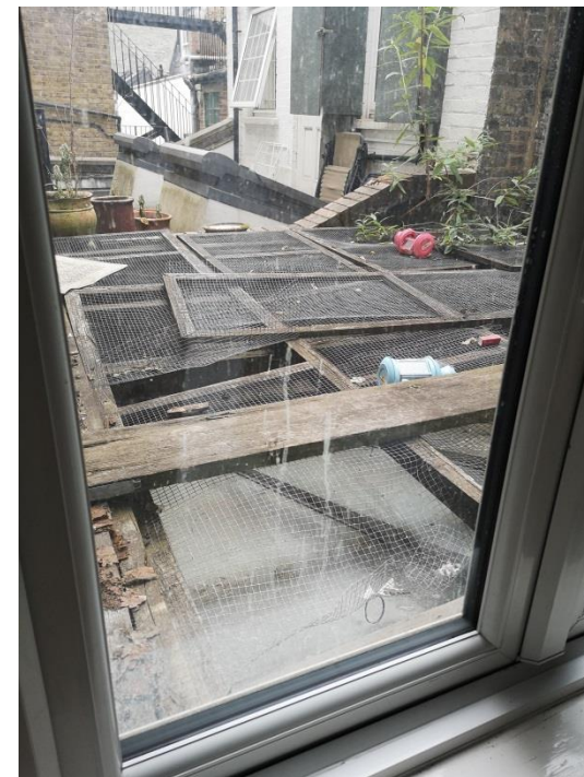
VIEW OF THE GLAZED ROOF ABOVE PIGEON PROTECTION
