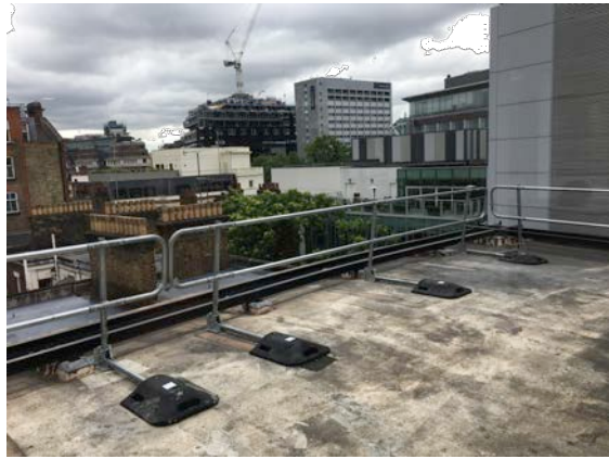
Photo showing the existing collapsible balustrade to the roof area
