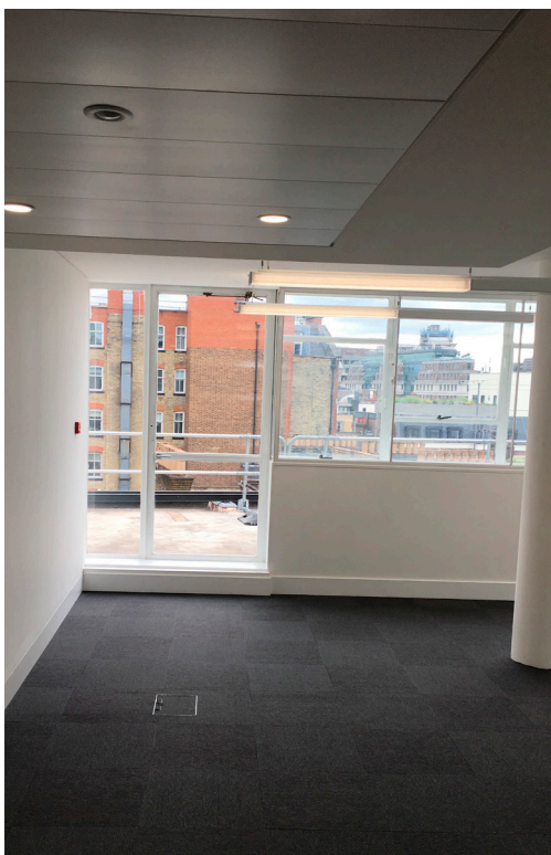
Views of the existing access door onto the roof
