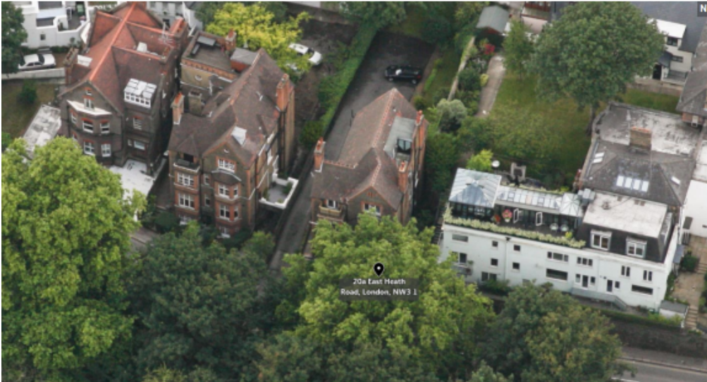
4. Front elevation and existing side dormer/terrace
