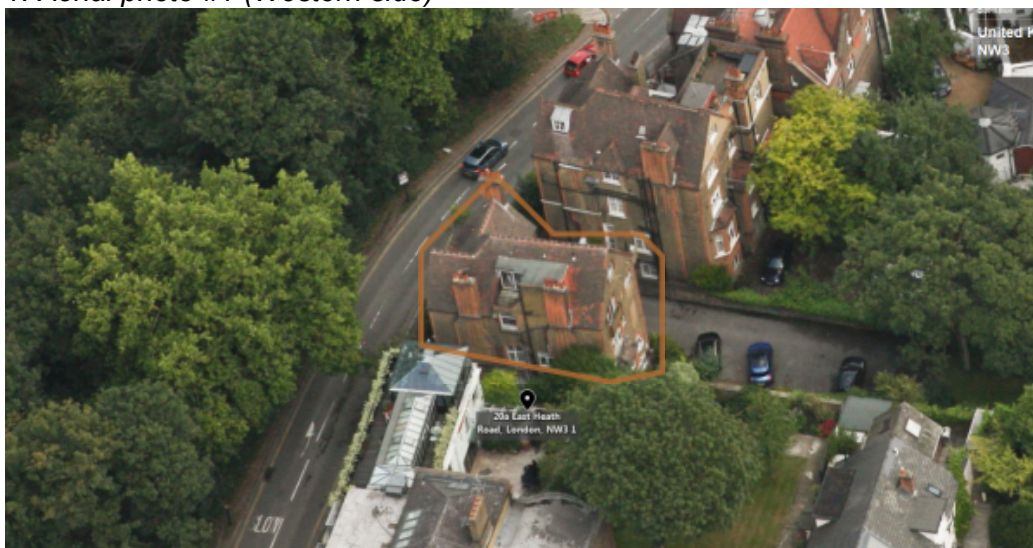
2. Aerial photo #2 (rear)
