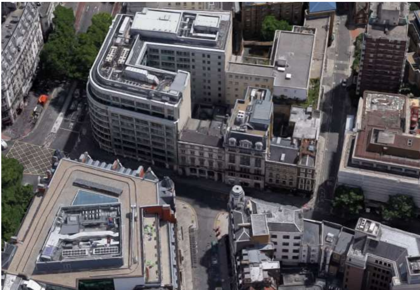
Figure 1: Aerial view of 212-214 High Holborn, from the north.
