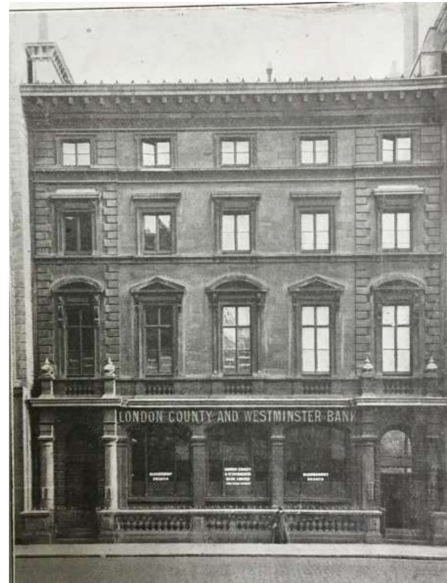
Figure 6: 1915 view of the London County and Westminster Bank.
