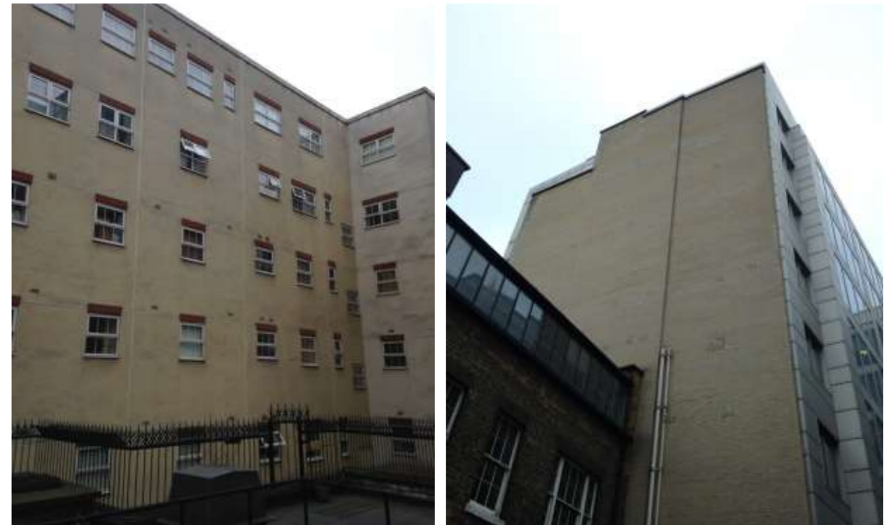
Figure 18: View south down Southampton Place towards the application site (top), rear element of No. 15 - 19 Newton Street (left) and the flank elevation of No. 215 - 222 High Holborn (right).
