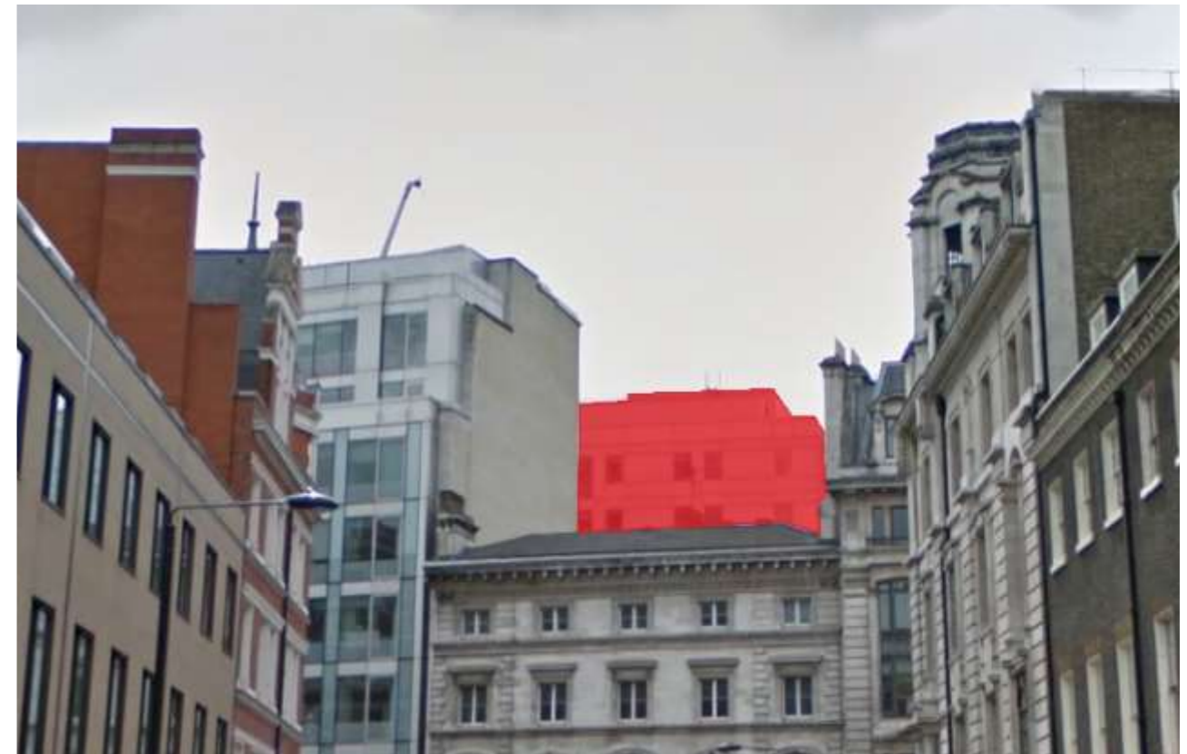
Figure 29: View towards the roof of No. 212 - 214 High Holborn, seen from Southampton Place. Nos. 15 -19 Newton Street highlighted in red.
