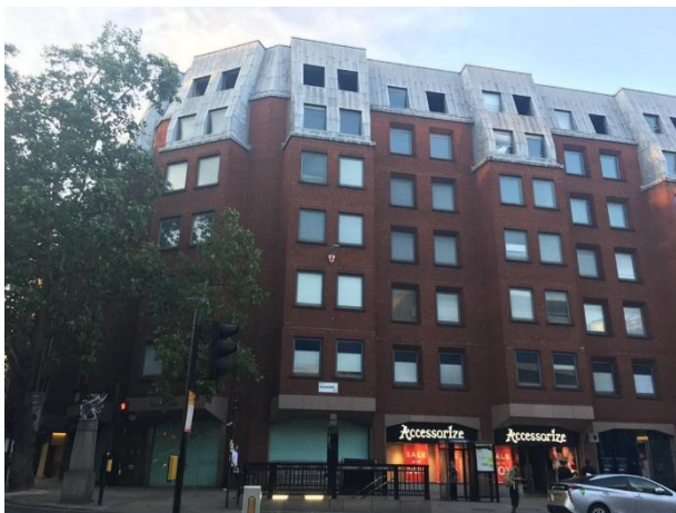
Photograph 1: Southern elevation of 150 Holborn
