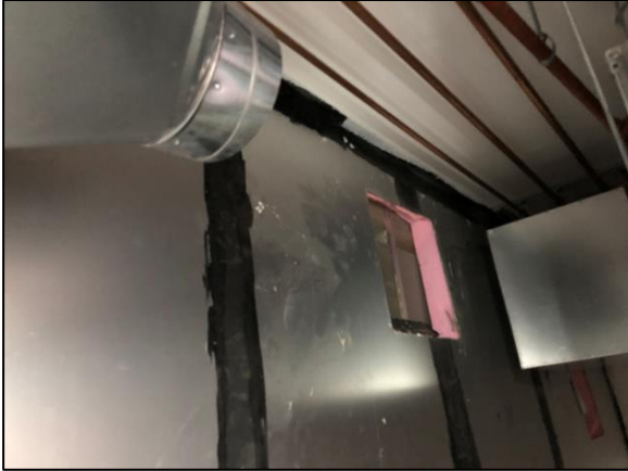
Photo.2.1. Existing louvers covered. Opening left for ductwork connection
