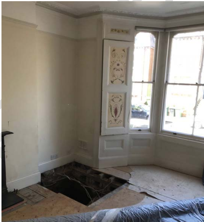
View of ground floor front room - No asbestos detected.
