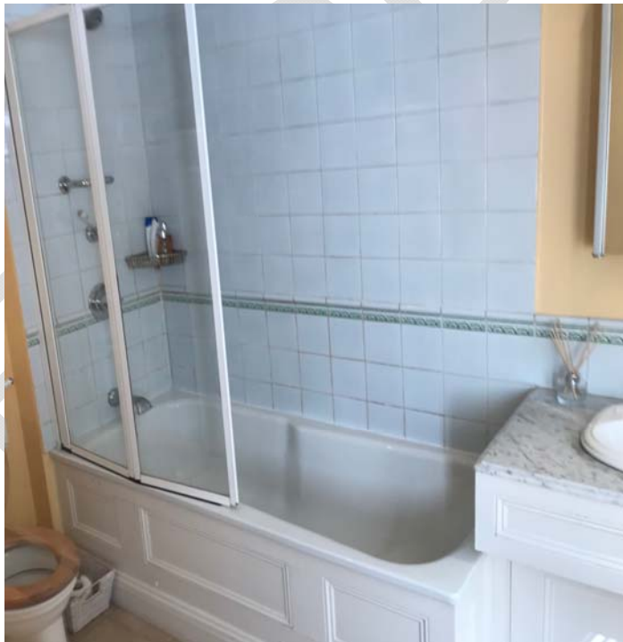
View of bathroom - No asbestos detected.
