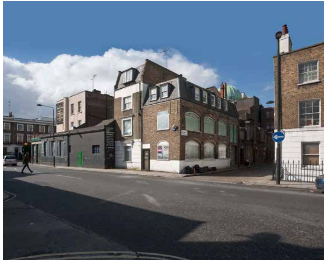
Existing view from Bayham Street
