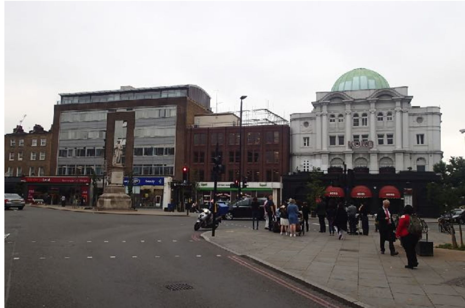
Existing building showing 3 storey addition to 48-56 Bayham Place under construction
