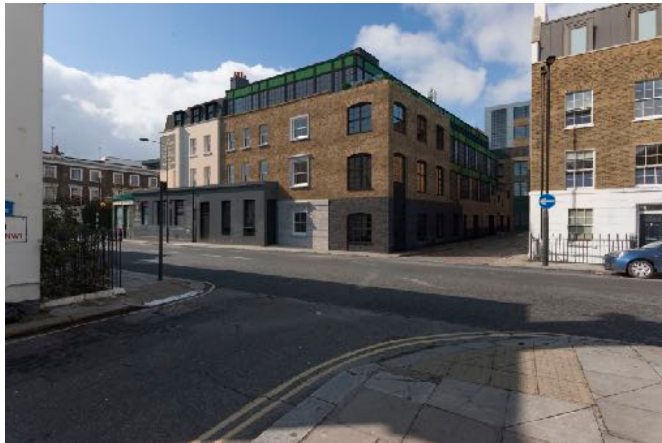
Proposed extension viewed from Bayham Mews showing Koko extension (currently under construction)
