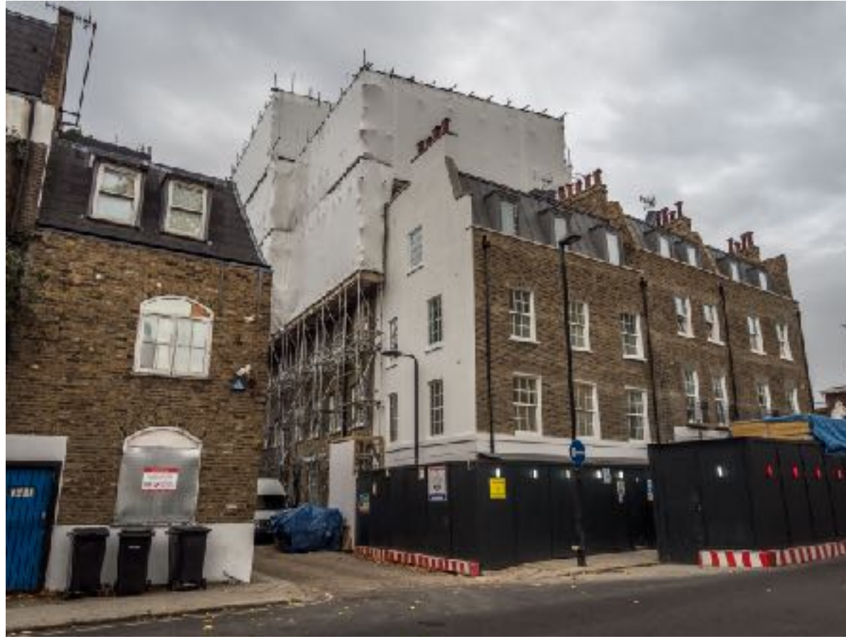
Entrance to Bayham Place showing extension to "Anders" building 48-56 Bayham Place
