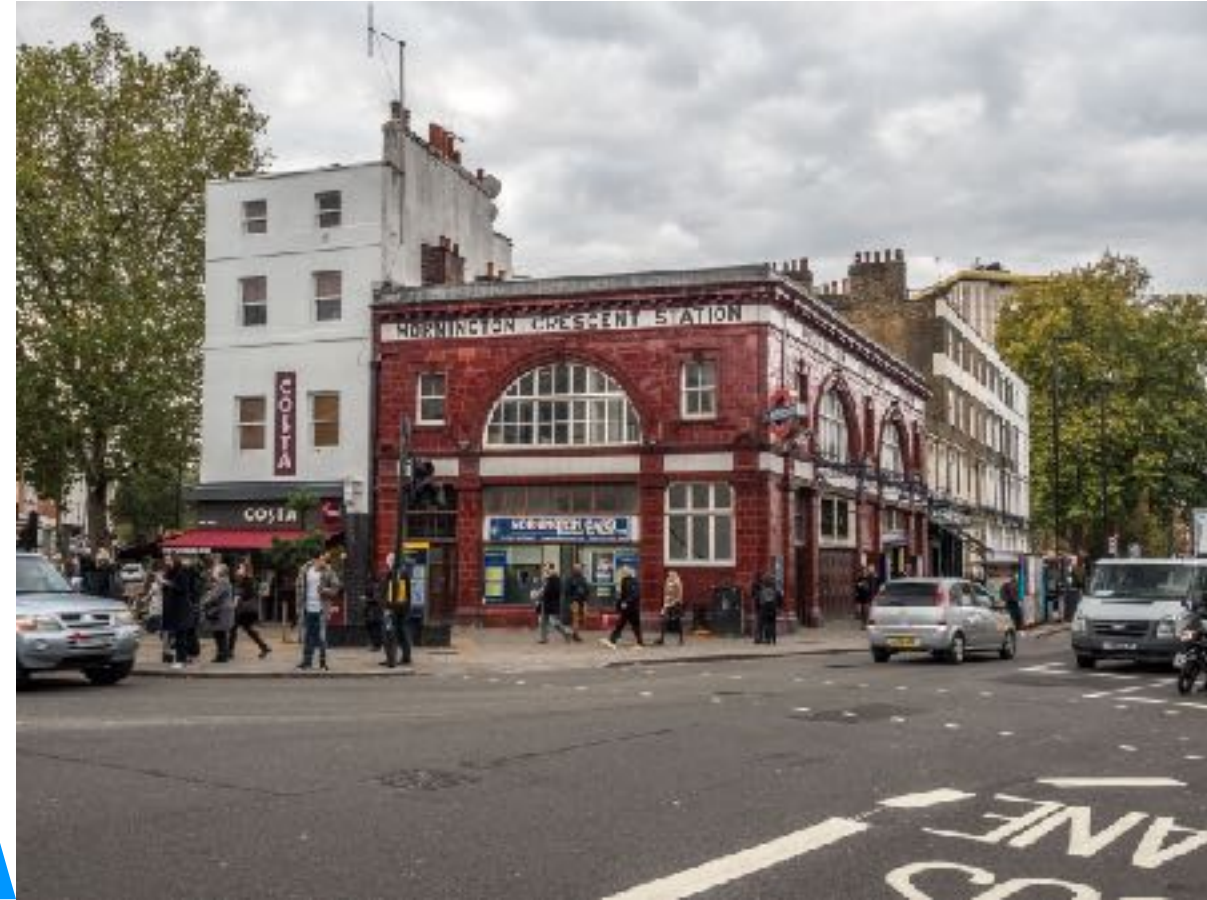
Mornington Crescent Tube Station
