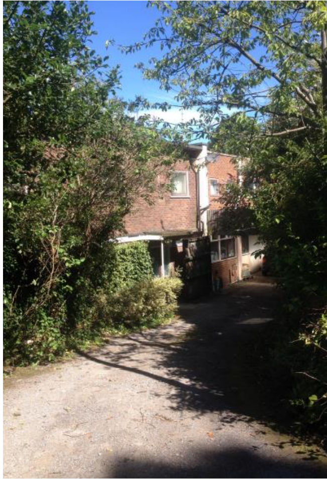
Existing building – View from Fitzroy Park entrance
