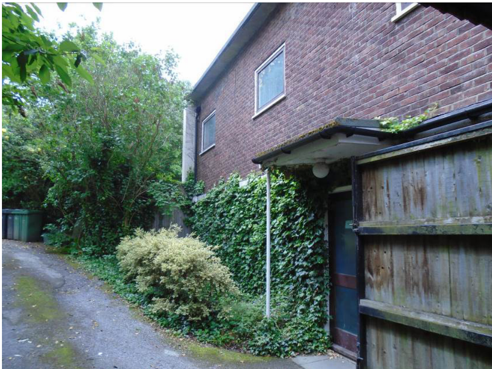
Figure 1: Front façade of no. 55
