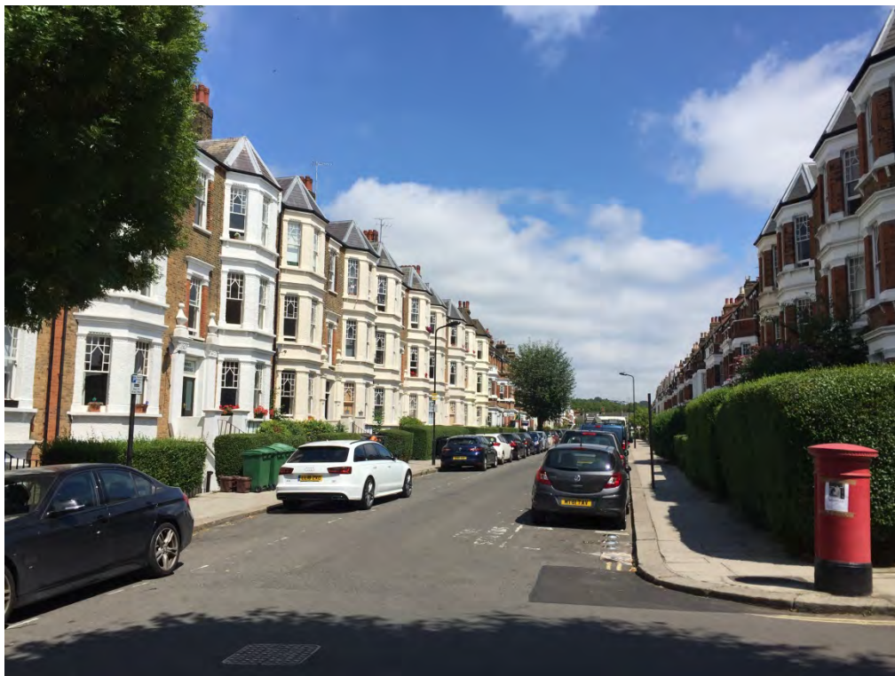
Plate 4: Mansion blocks of Gondar Gardens to the north of the Site, entered on the Camden local list.
