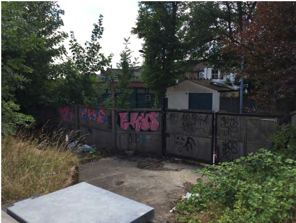
Plate 6: Existing hoarding along Gondar Gardens frontage, viewed from within the Site.
