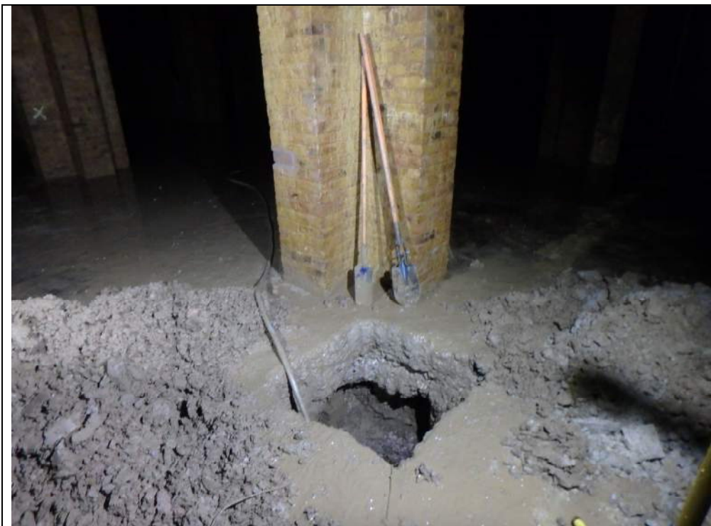
Plate 8: General view of trial pit 1.
