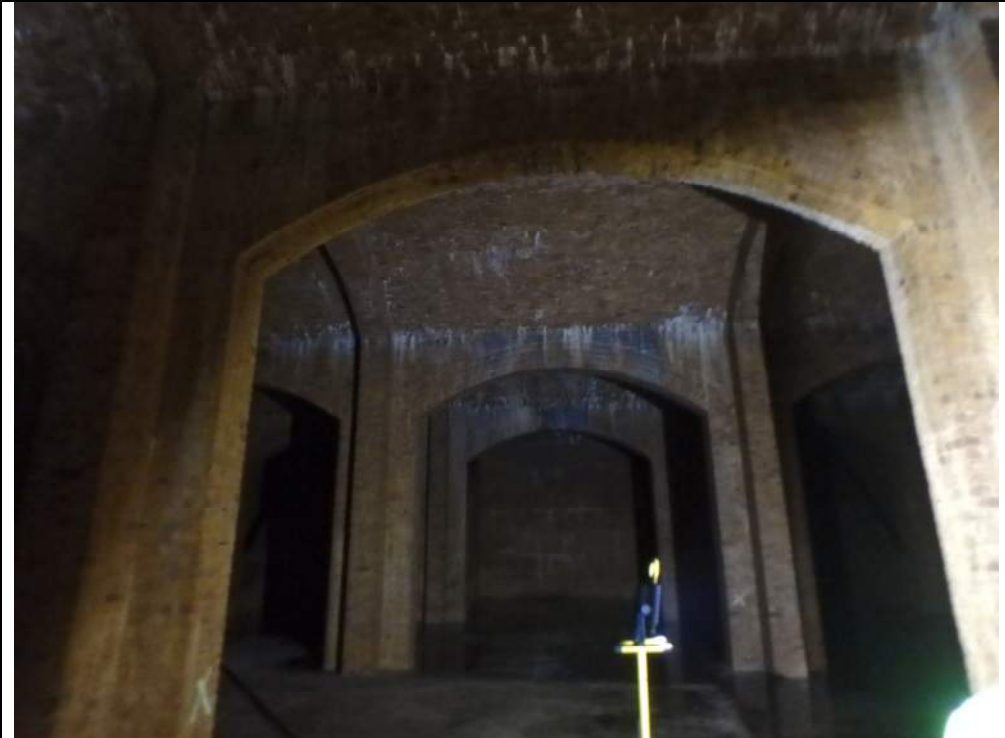
Plate 1: General view of brickwork.
