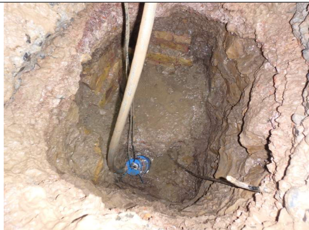
Plate 12: View inside trial pit 2.
