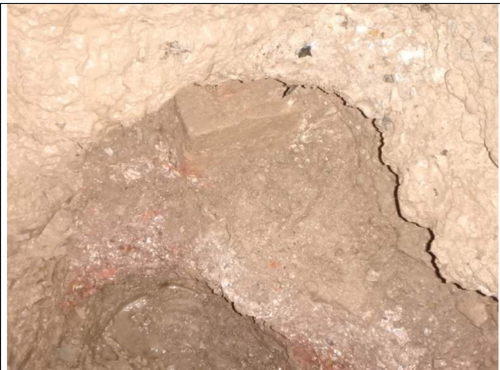
Plate 10: View of brick corbel sitting on concrete pad in trial pit 1.
