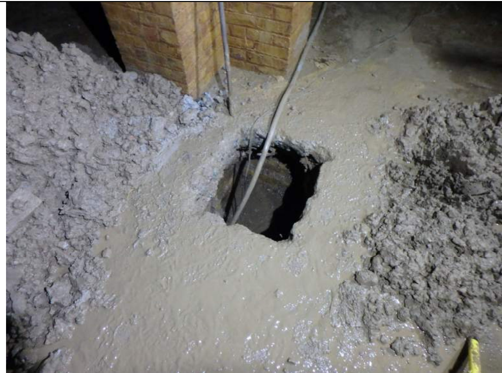
Plate 11: General view of trial pit 2.
