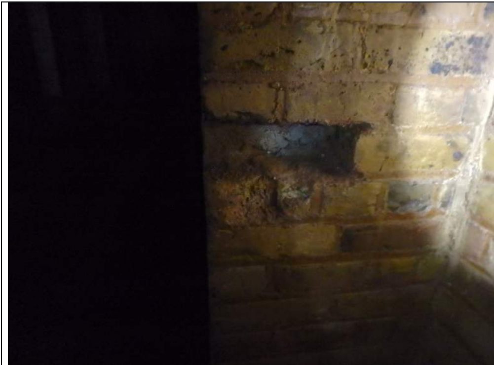
Plate 5: Column where brick & mortar samples B5 & M5 were extracted.
