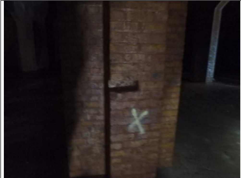
Plate 3: Column where brick and mortar samples B2 & M2 were extracted.
