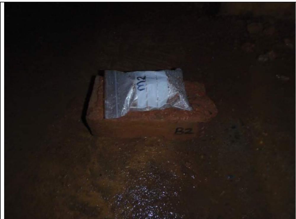
Plate 2: Brick and mortar samples B2 & M2 extracted from column.
