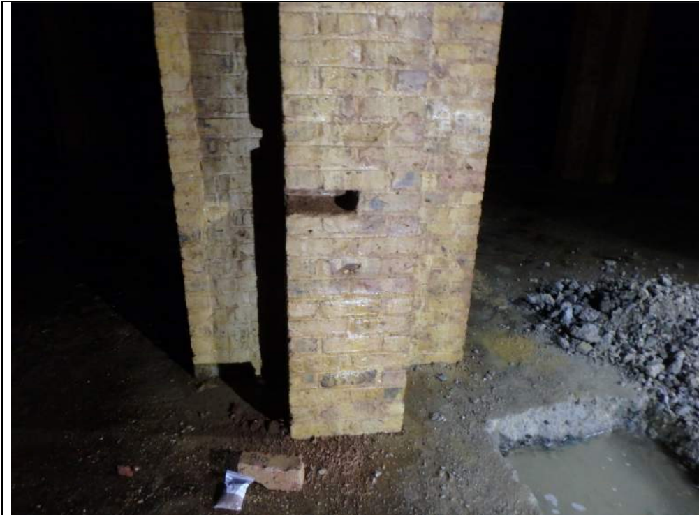
Plate 7: Column where brick and mortar samples B10 & M10 were extracted.
